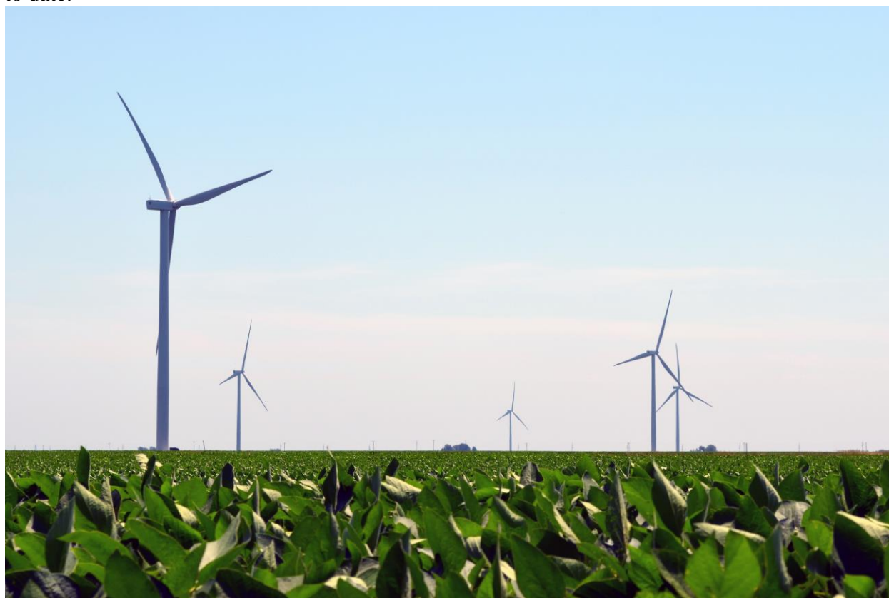
Photo: Several of the 53 turbines that make up the Bishop Hill III Wind Energy Center.
