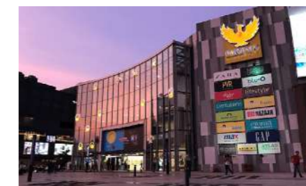
Phoenix MarketCity, Bengaluru 0.31 msft Leasable area Addition of retail space to Phoenix MarketCity Bangalore
