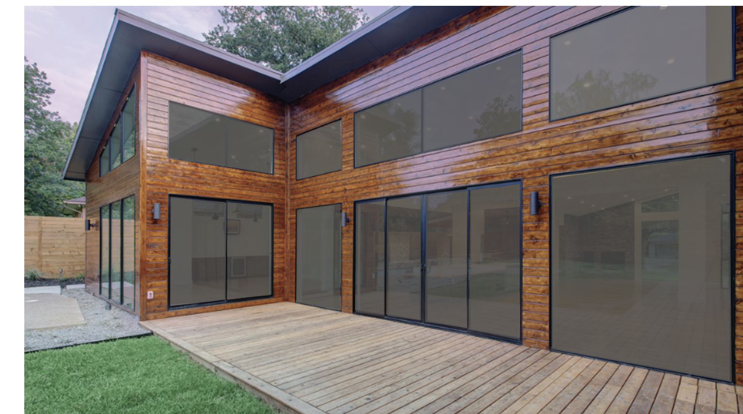
ALUMINUM FRAME EXTERIOR WINDOW AND DOOR COMPANY: ANDENSEN FRAME LRV: 4.51 GLAZING LRV: 40
