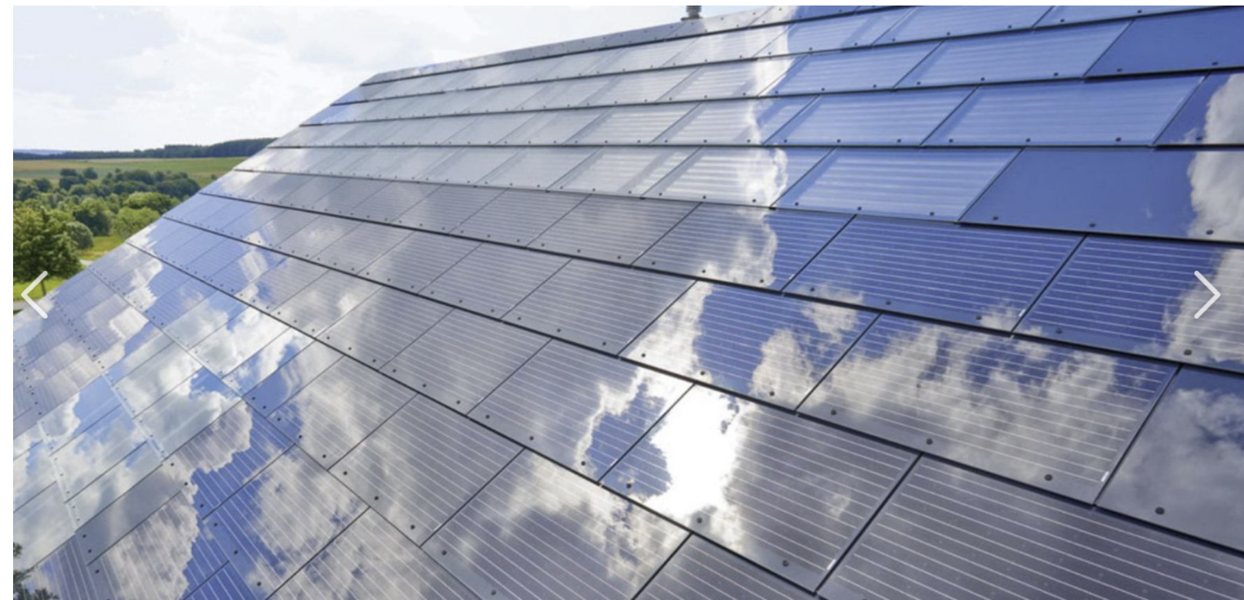
SOLAR PANEL ROOF TILE - TESLA LRV: +/-10.0
