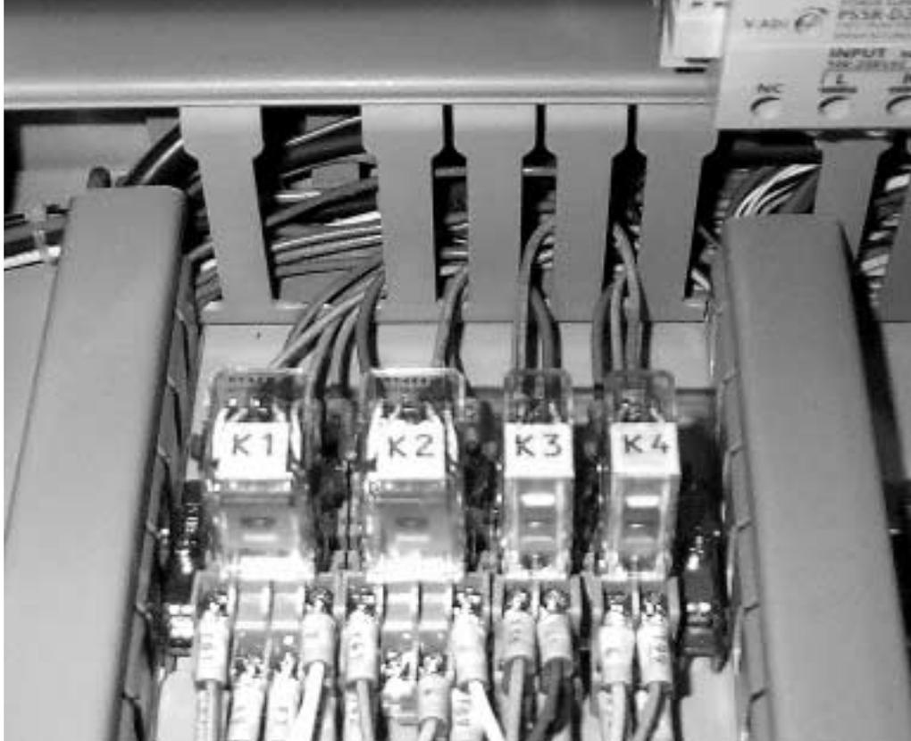
**K1 (Quartz Lamps Relay 4 Pole 120 volts AC)** - This relay is used to signal the optional Quartz Lamp Flash Cure Units to cycle up to the pre-selected output power setting for flashing of garments.
