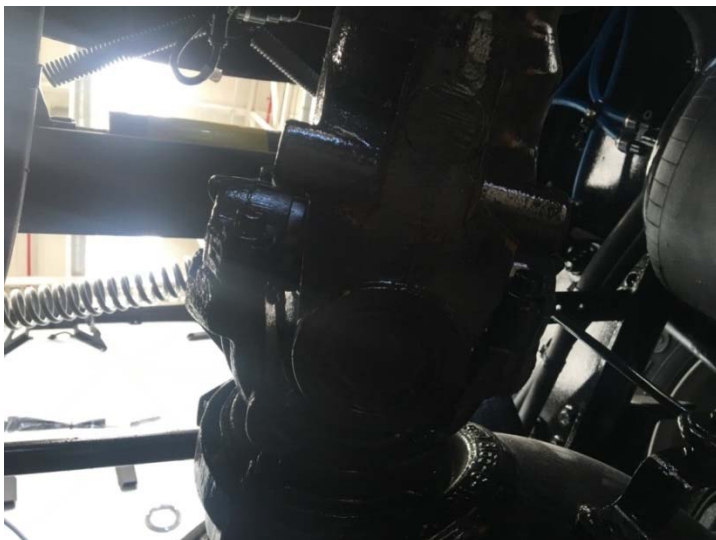
Figure 16 – Yolk Bolt Installation
