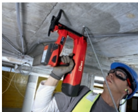
Threaded rod attachments to concrete
