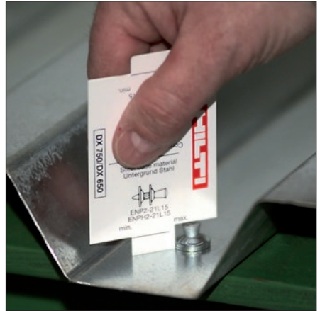
Checking the standoff of an ENP2 roof deck fastening with a plastic gauge
