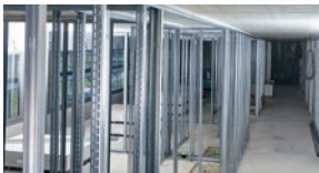
Drywall tracks to concrete and steel
