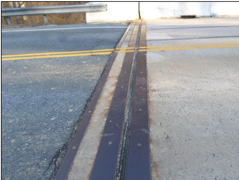
22. Typical roadway joint (east joint shown)
