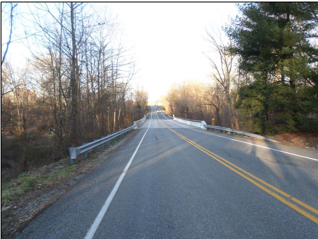
2. East Approach Looking West
