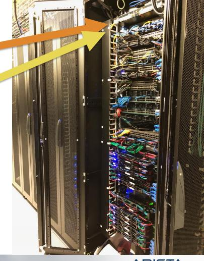
Reducing the length of the cables now has a significant effect on total latency
