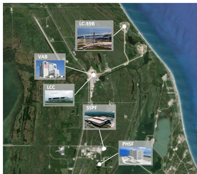
Figure 7-1: Aerial Overview of KSC Facilities
