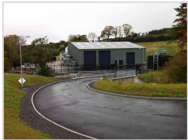
New Kilsellagh Water Treatment Plant commissioned in June 2010.
