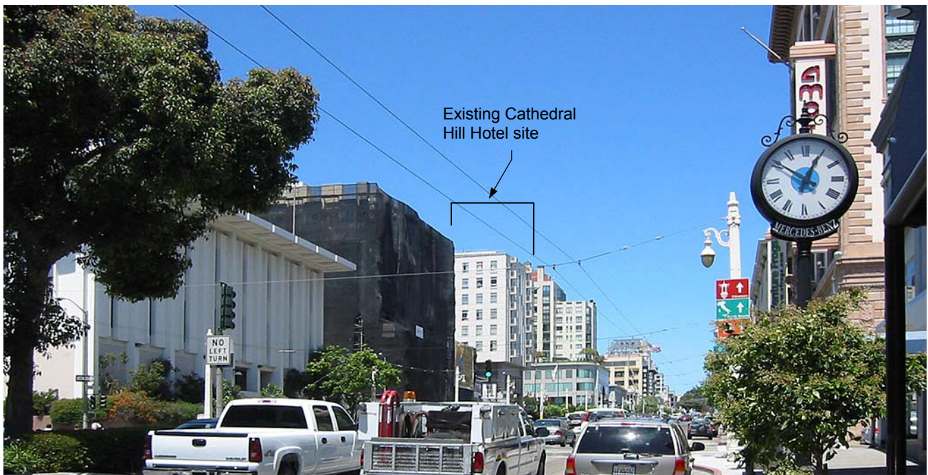
Existing View—looking north along Van Ness Avenue from between Ellis and O’Farrell Streets toward the existing Cathedral Hill Hotel on Van Ness Avenue
