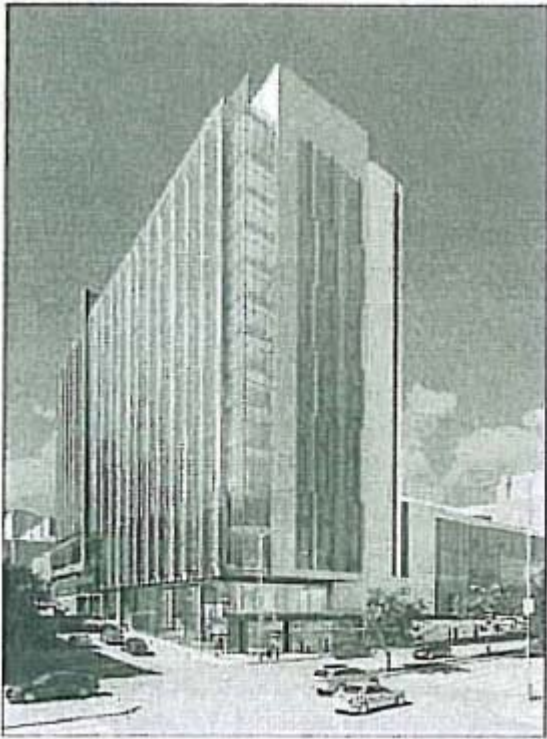
Figure 5: CMPC Cathedral Hill Hospital as seen from Van Ness Avenue at Geary Boulevard From: California Pacific Medical Center 2008 Institutional Master Plan; http://www.rebuildcpmc.org/assets/08IMP_CPMC.pdf
