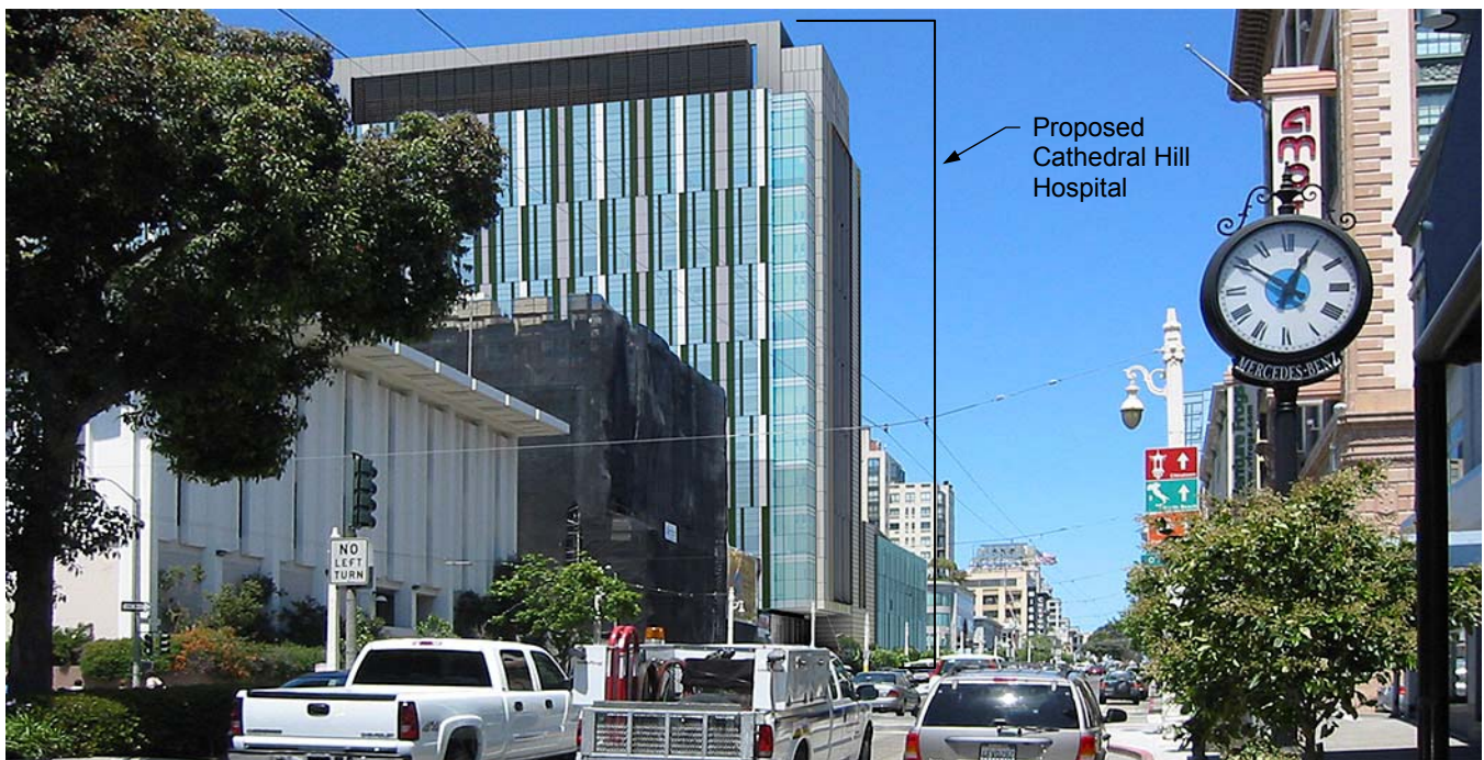
Proposed View—looking north along Van Ness Avenue from between Ellis and O’Farrell Streets toward the proposed Cathedral Hill Hospital on Van Ness Avenue
