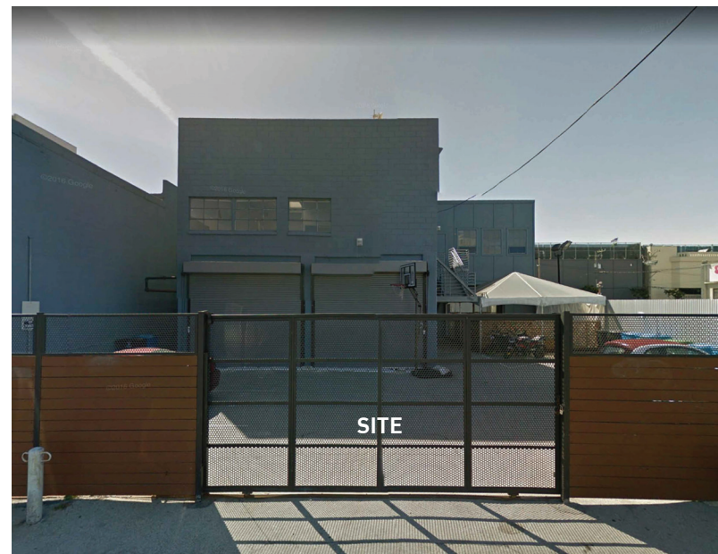
8. FREELON STREET LOOKING SE
