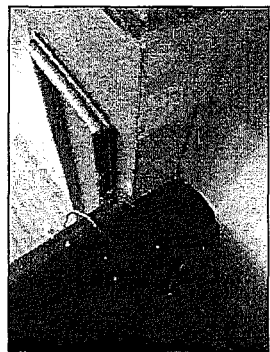
PHOTO 2: HISTORIC HANDRAIL TO BE SALVAGED AND RETURNED TO OWNERS. USE CAUTION WHEN REMOVING HANDRAIL FROM AROUND PROSCENIUM.
