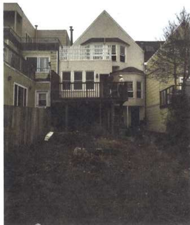
REAR FACADE OF SUBJECT PROPERTY
