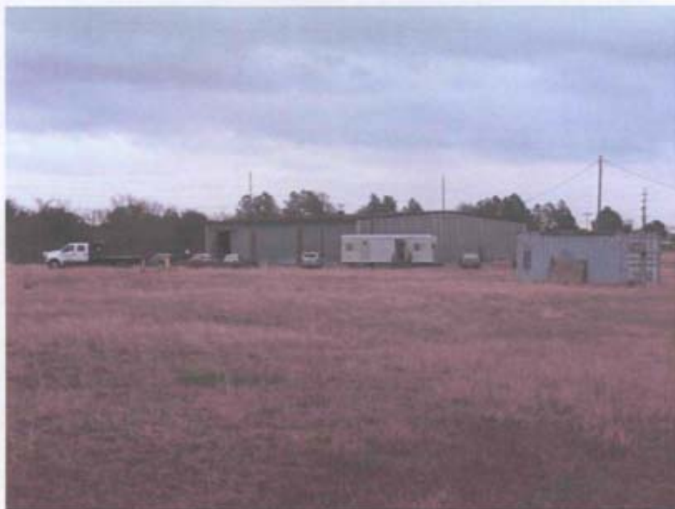
A metal warehouse used for storage, located on the Peak Oil Co. portion of the Site.
