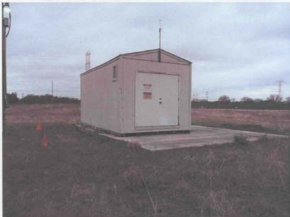
The air sparging system building located north of the wetlands at OU4.
