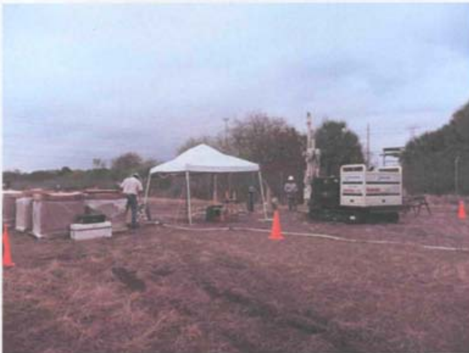
The organic substrate injection being completed during the site inspection.
