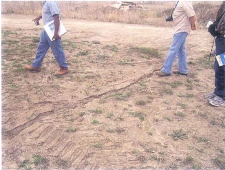
Sludge Lagoon Cover – Minor Erosion Gully on east side
