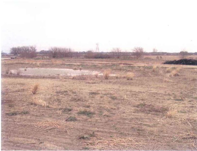
Sludge Lagoon Cover – Ponding in Low Spot on South-Center of Lagoons
