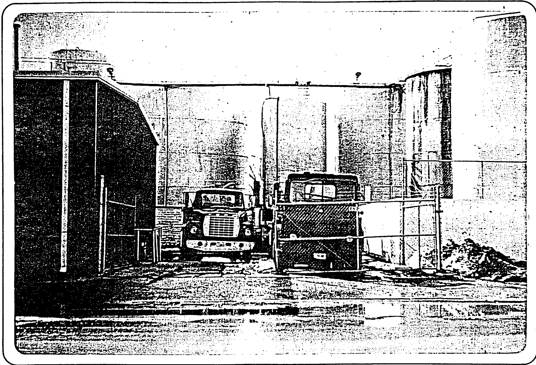
Figure 2.4 Photograph of some of the tank farm at Capitol Oil, taken March 22, 1985.
