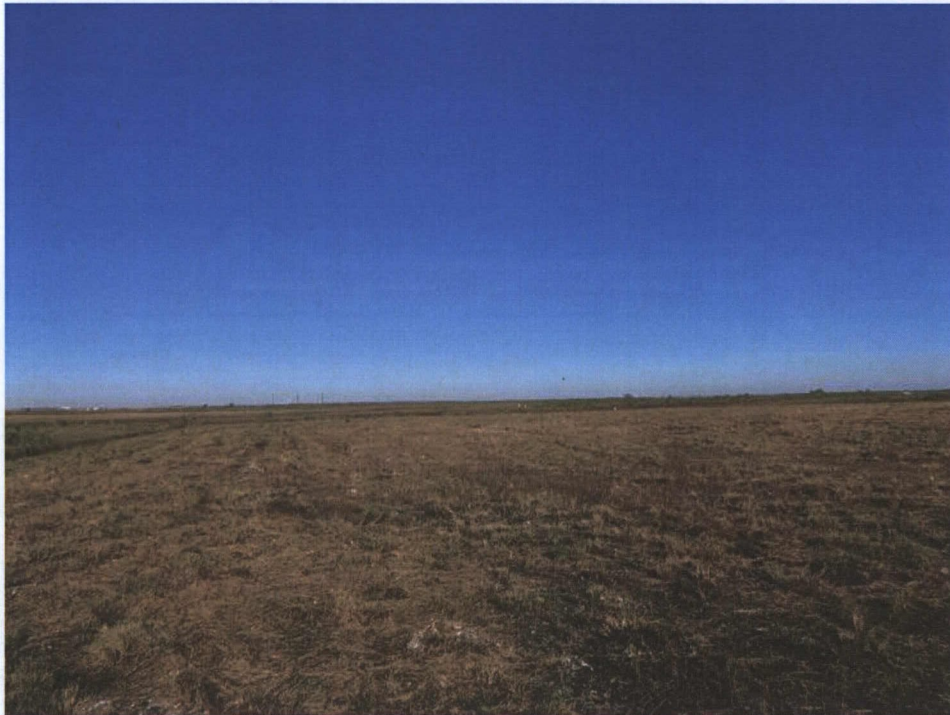
Cap on the former surface impoundment area, facing northeast.
