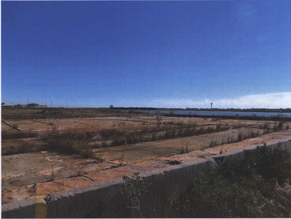
Former AST Tank Farm in South Area of the Site.
