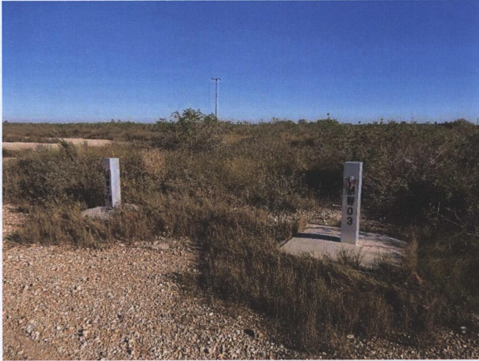
Locked and marked monitoring wells MW 03 and MW 24B.
