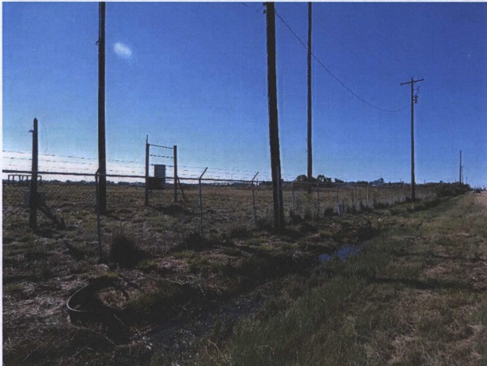
Fence on perimeter of South Area of Site.
