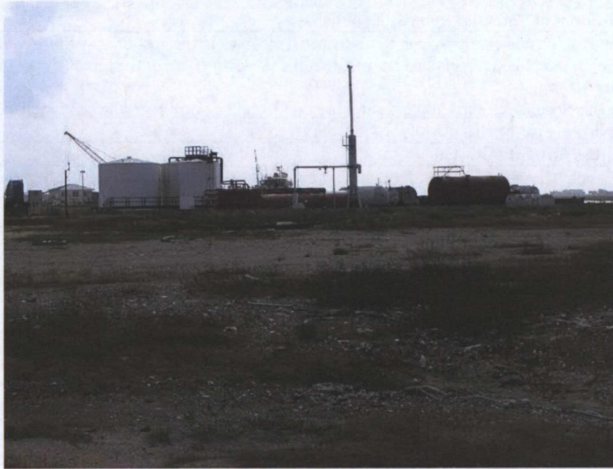
Tanks on the Site.
