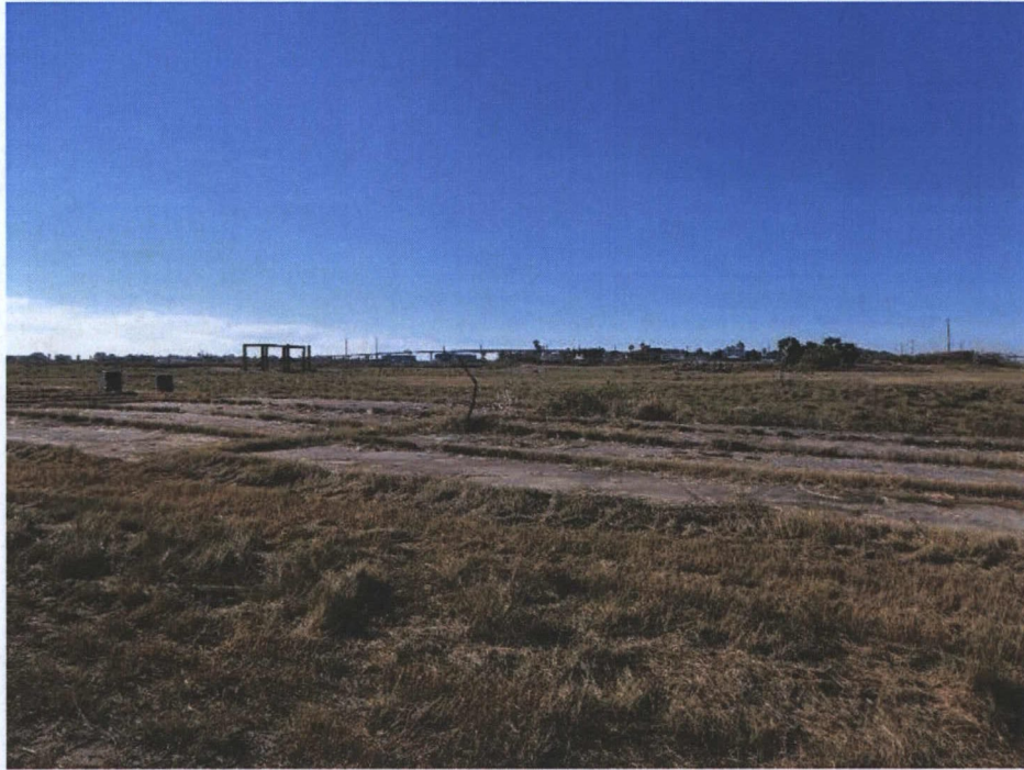
Concrete pad in South Area of the Site.
