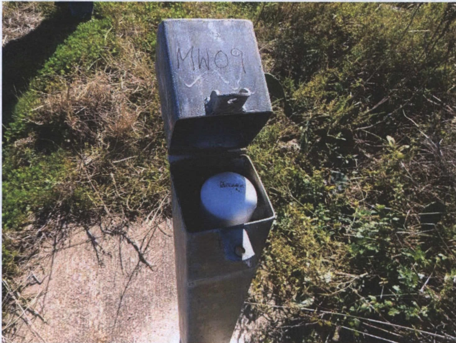
Interior of MW 09.
