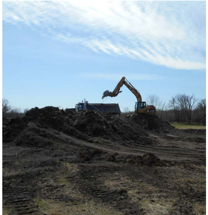
Cleanup of Chat Pile CP009.
