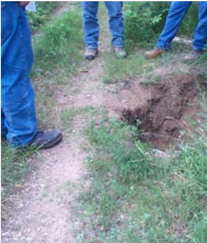
OU1 O&M activities include repairing dike collapses, as shown above.
