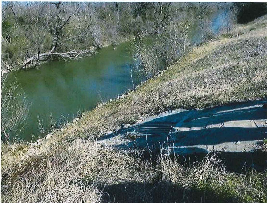
Drainage corrugated metal pipe outfall from North Property to Leon River.
