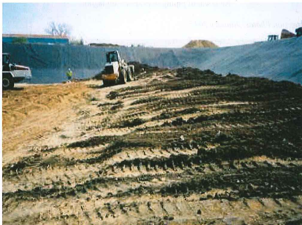
Waste being placed in containment cell.
