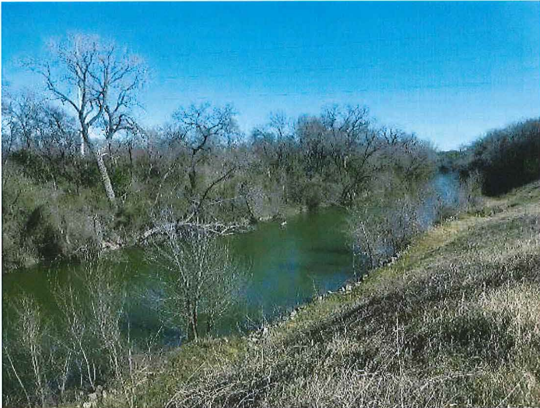
Leon River bank with articulated concrete blocks.
