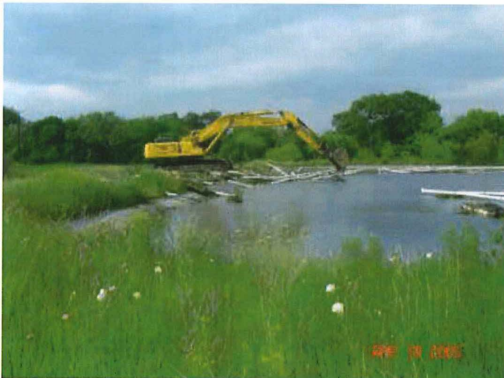
Removal of piping in evaporation lagoon.
