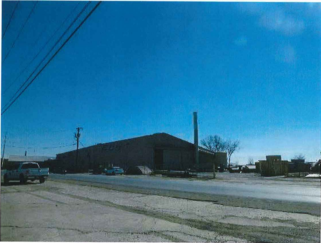
Engineered Composite Systems on OU2 property.
