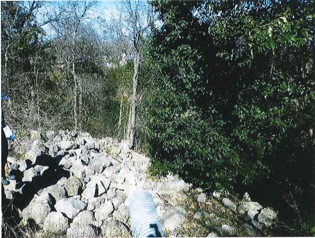
Drainage corrugated metal pipe outfall to Leon River.
