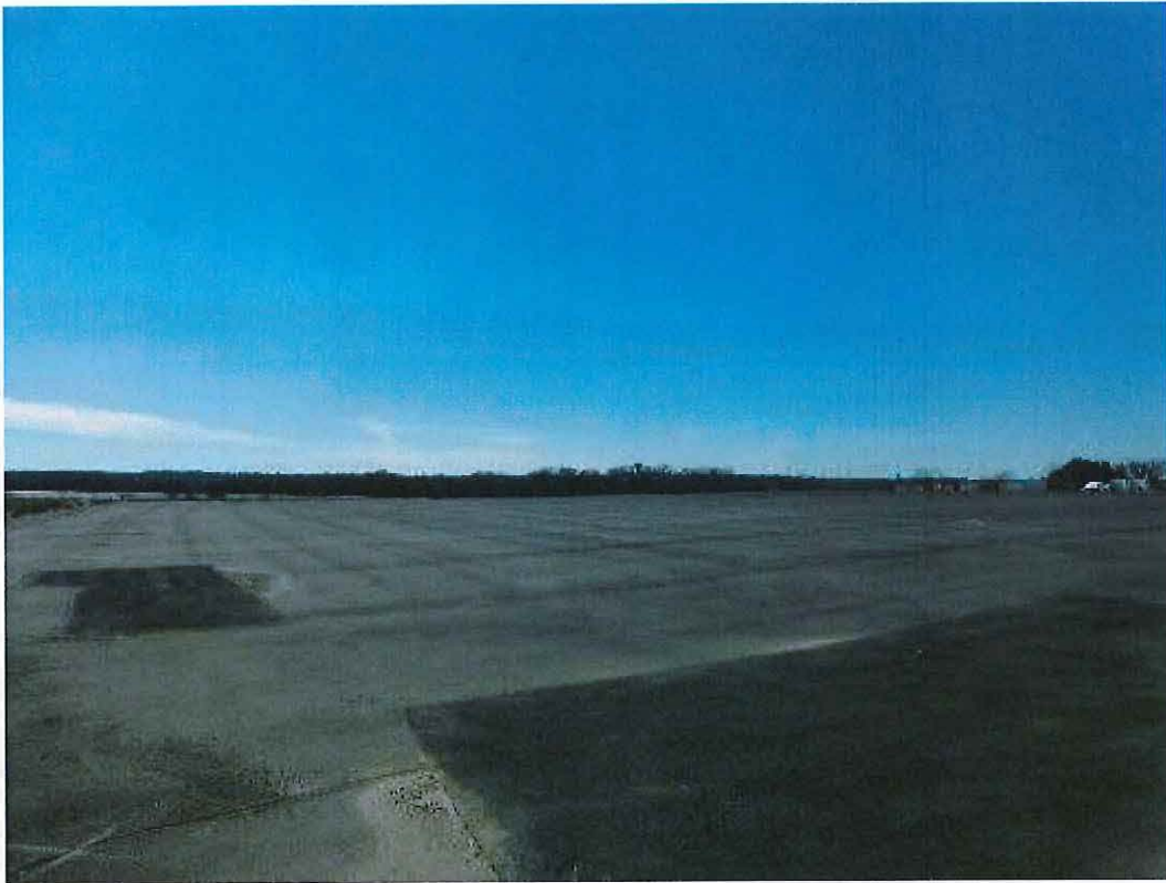
MatCon cover, facing southwest.
