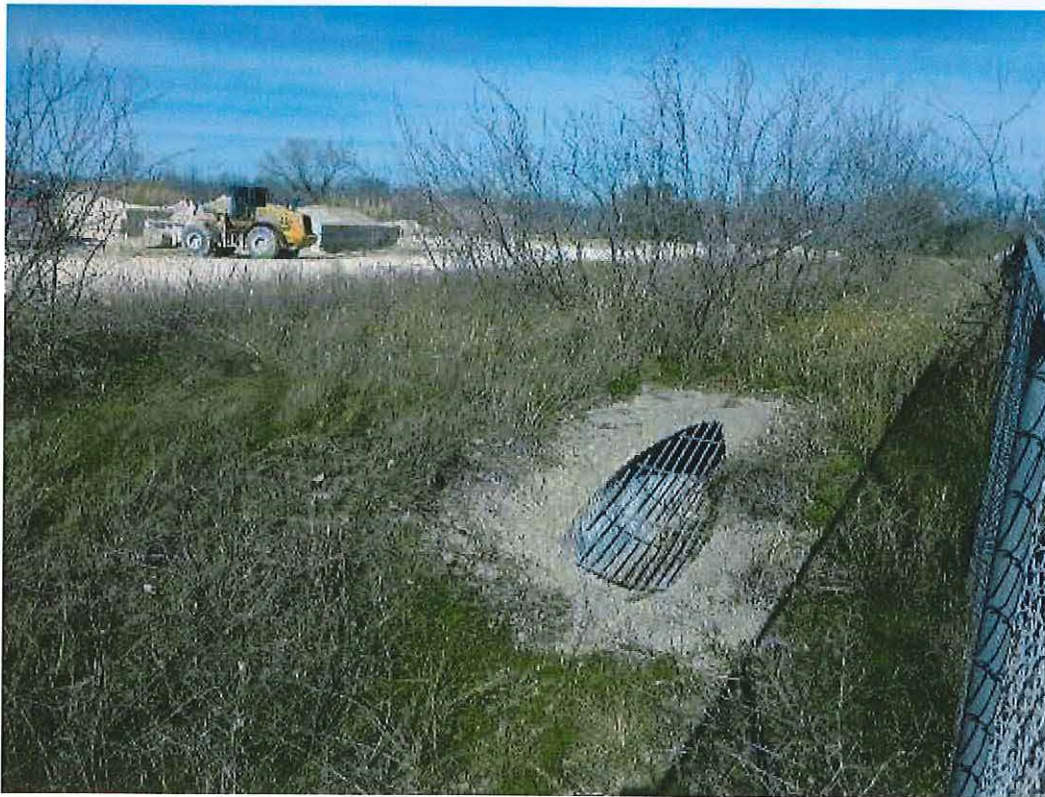
Drainage corrugated metal pipe west of Cemetery Property.
