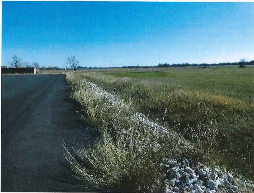
Surface water drainage south of MatCon cover.
