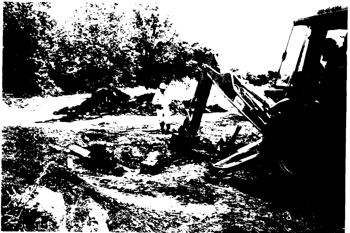
Photograph No. 24 Area D Looking East, Continued East Sump Excavation
