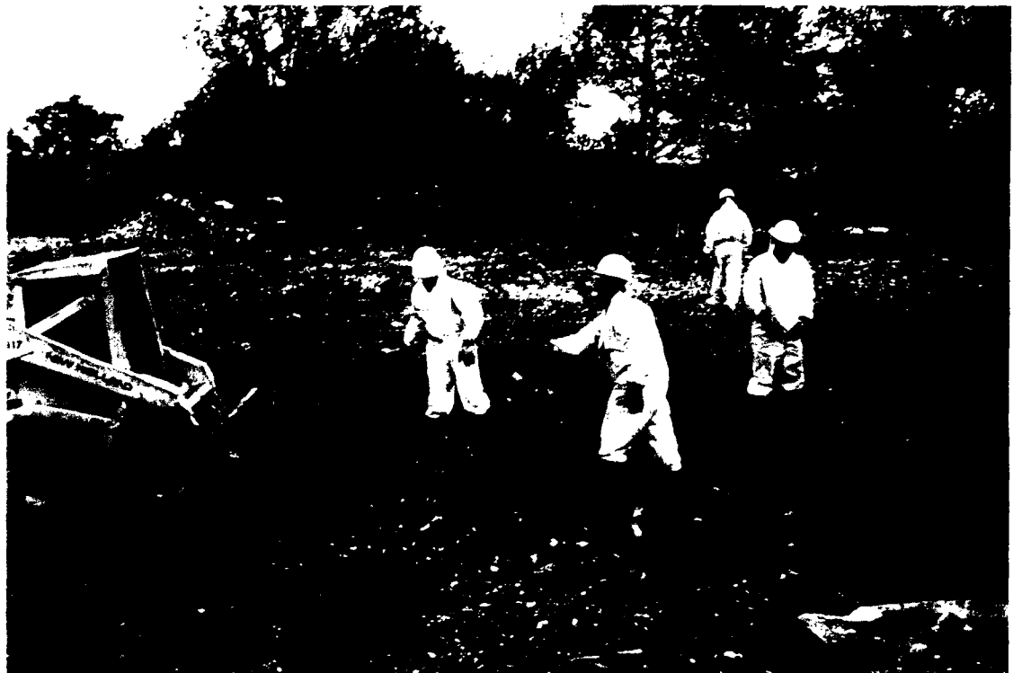
Photograph No. 32 Area C Looking North, Continued Hand Picking (Concrete Slab in Foreground)
