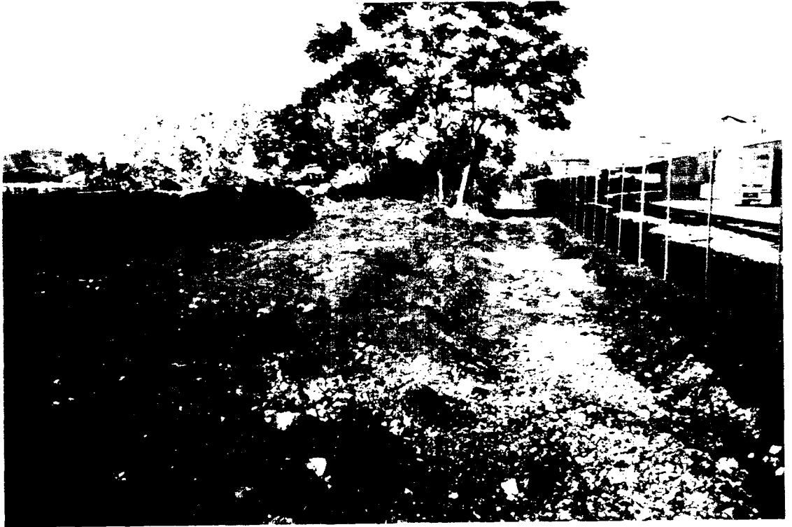
Photograph No. 7 Area G Looking West, After Removal was Completed
