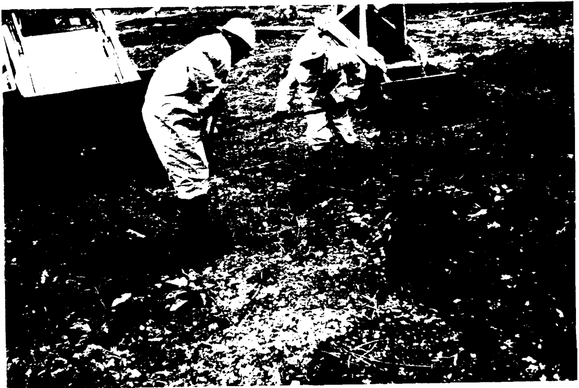
Photograph No. 34 Area B Looking South, Hand Picking Residual Asphalt
