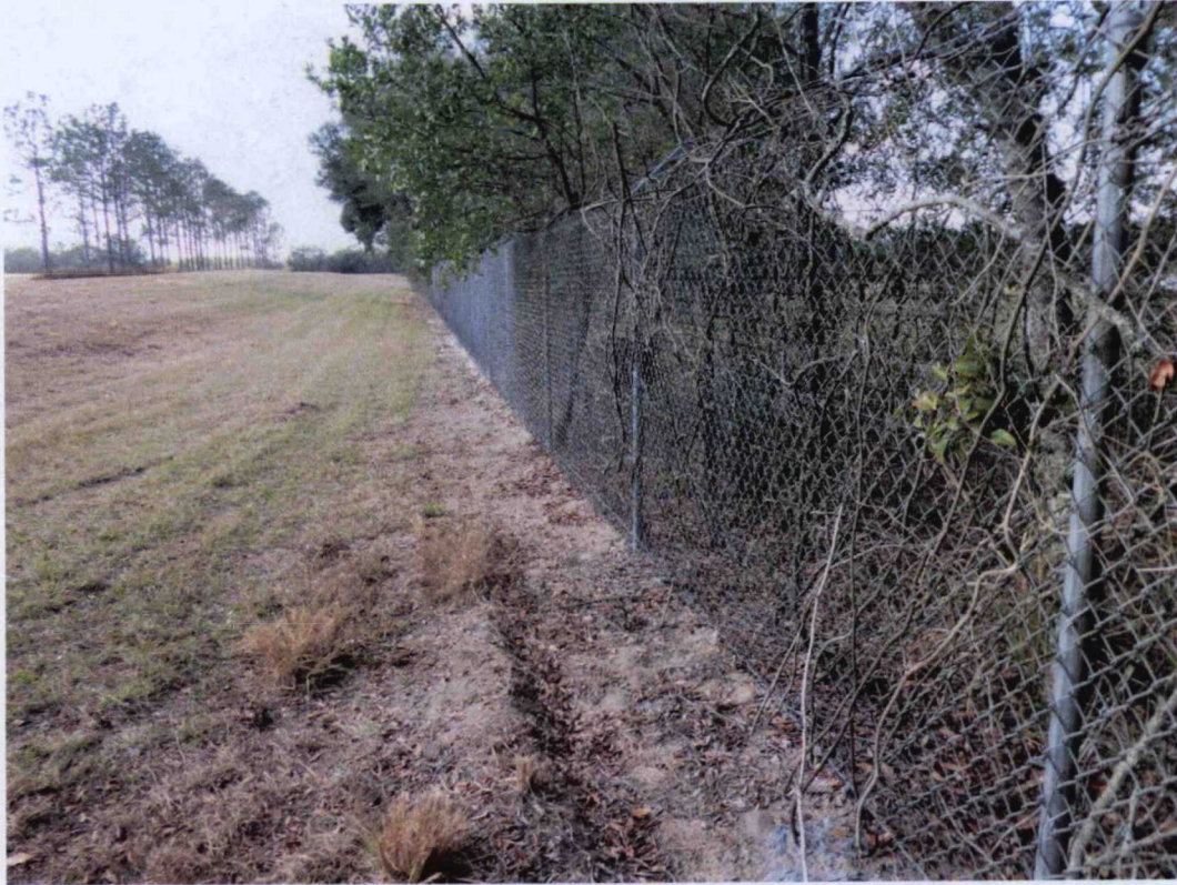
Fencing around the county landfill complex
