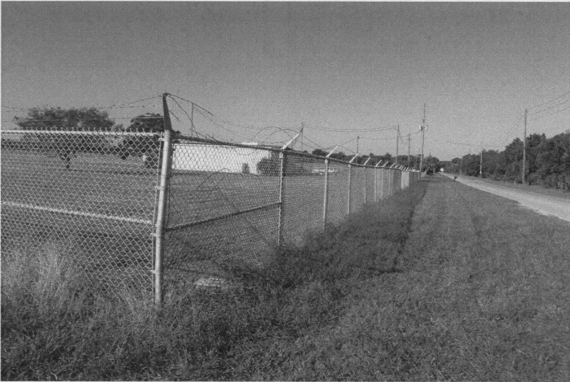
Fence line around south landfill along Anclote Road.
