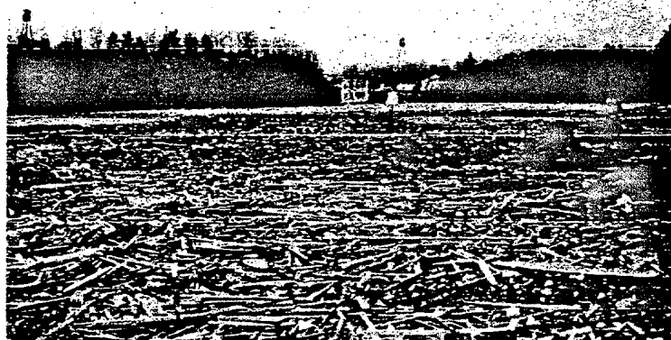
Figure 13. View upstream (to west) off north end of Rogers Island, Fort Edward, showing upstream edge of mass of debris that washed down from the remnant deposits north of the former Fort Edward Dam and clogged the Fort Edward terminal (marked by parallel diagonal lines at bottom of Figure 11). (NYS DEC photo taken in April 1974.)
