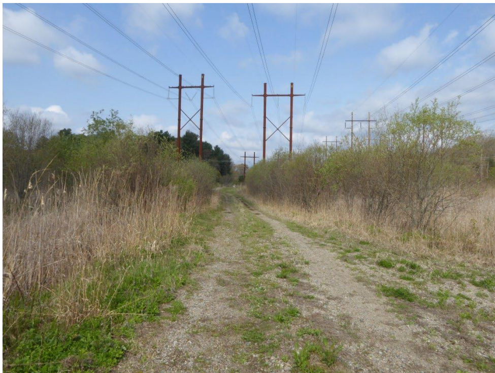
Access road for National Grid utility easement
