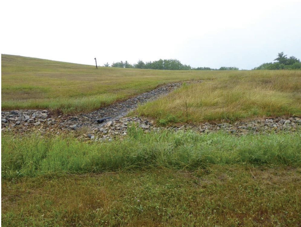
Outlet pipe on Landfill Area 3
