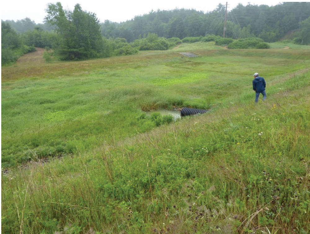
Outlet structure into the retention basin
