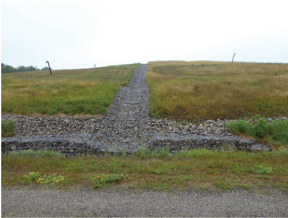
Gabion-lined letdown channel and retaining structure on Landfill Area 3
