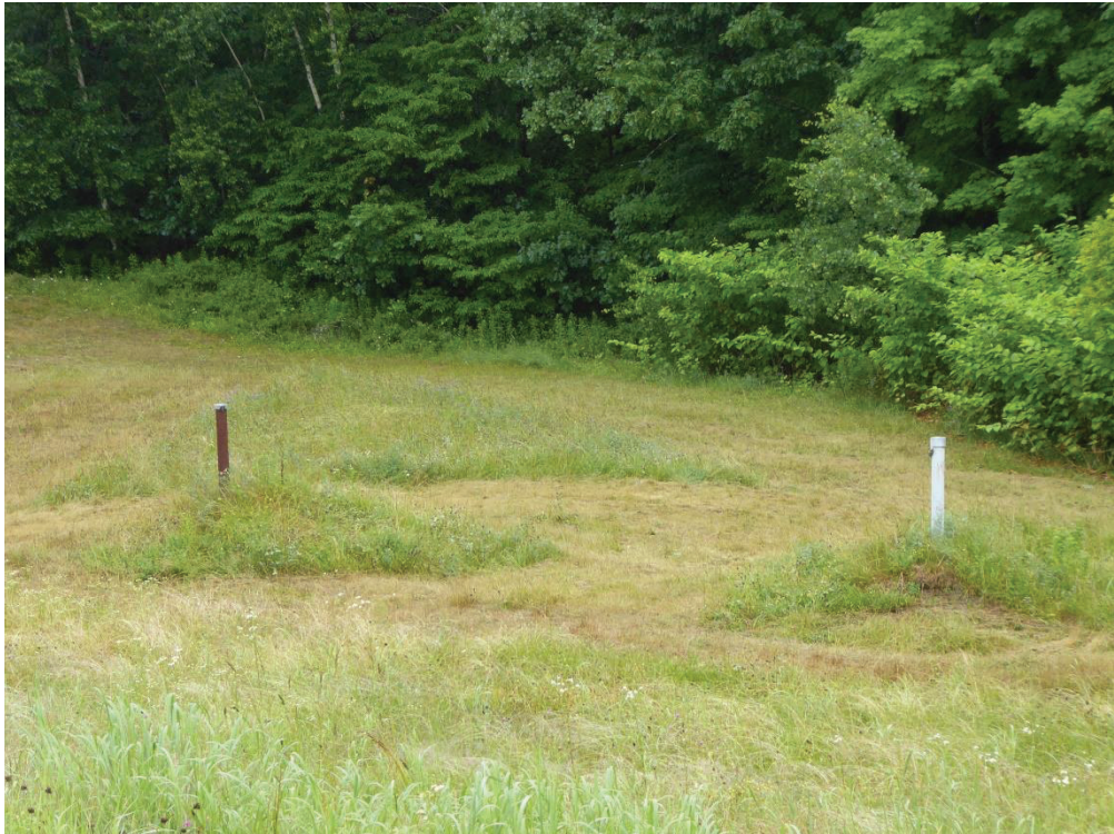
Groundwater monitoring wells
