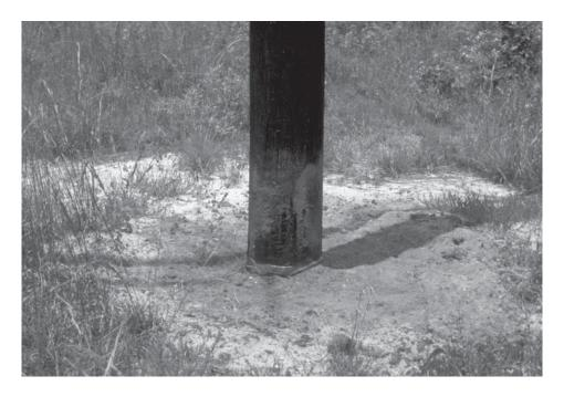
Fig. 4. Wild pig rub on a telephone pole.
