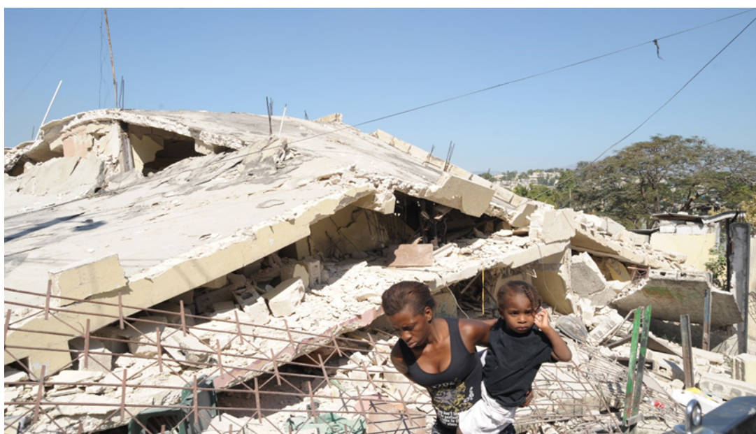
Figure 4: The aftermath of the 2010 magnitude 7.0 earthquake in Haiti
