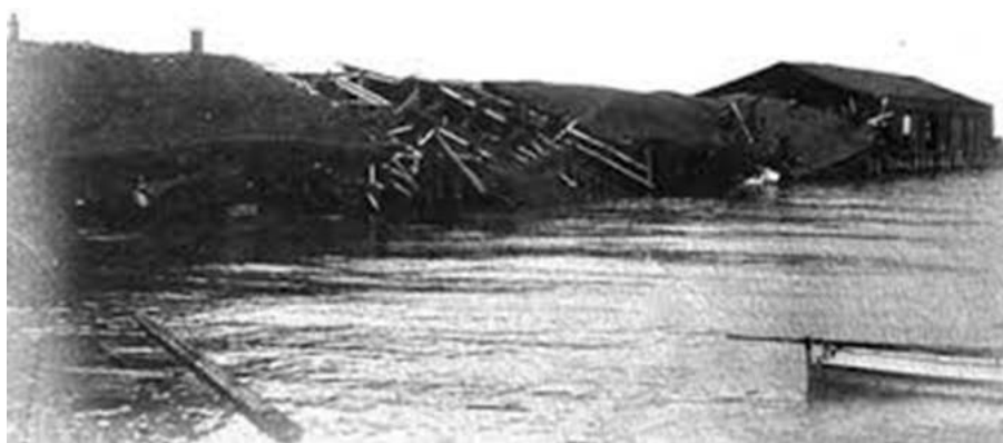
Figure 42. Historical photograph of the Pacific Lumber Company dock at Fields Landing that collapsed from liquefaction triggered by the 1906 San Andreas fault earthquake. (Image reproduced from Dengler, 2008, her Figure 8.)
