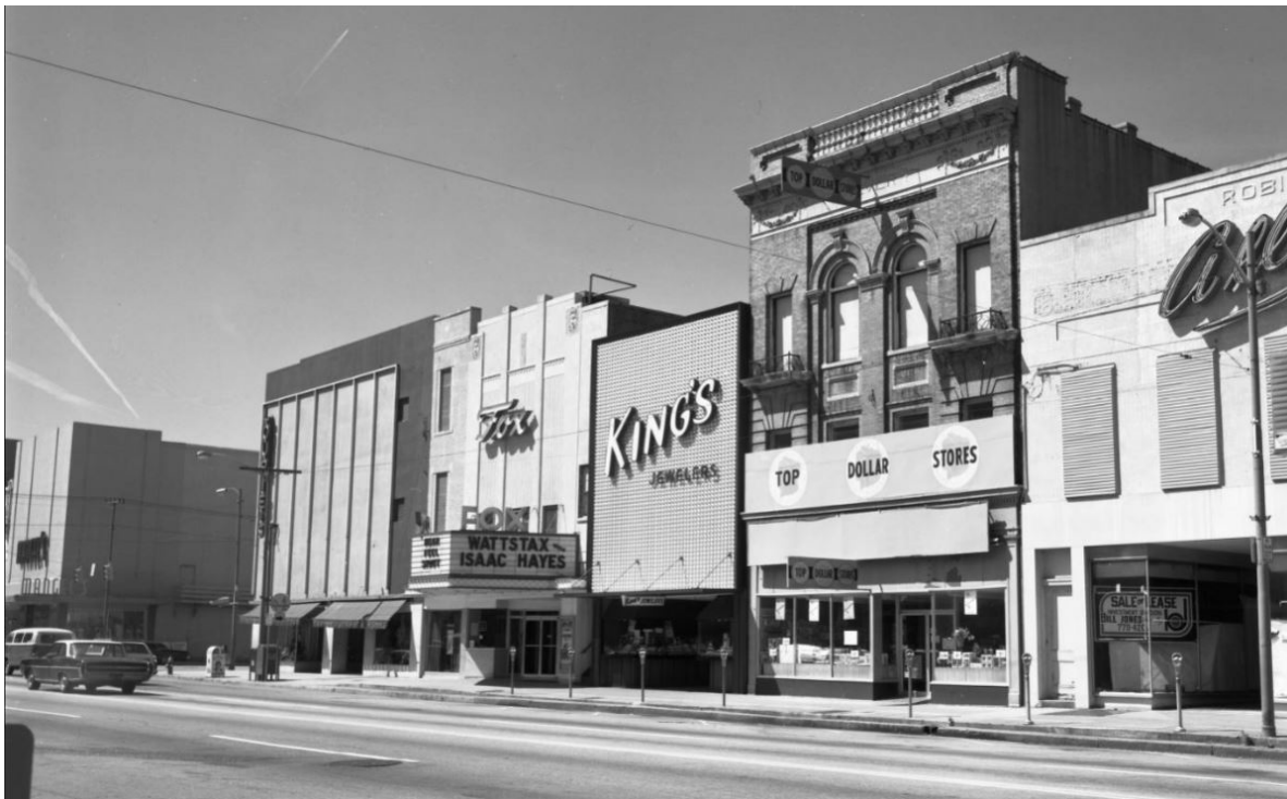
Figure 3.30. 1600 block of Main Street with its new Modernist facades, photograph by Russell Maxey, 1978. Russell Maxey Photograph Collection, RCPL.
