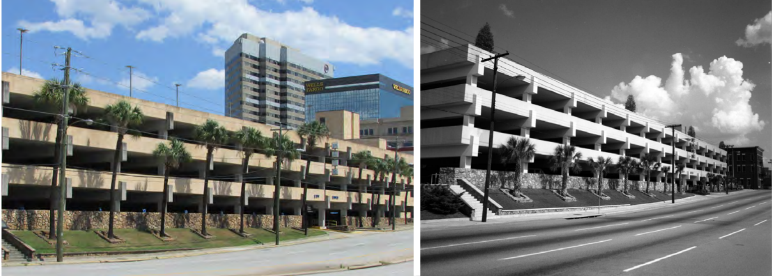
Figure 3.27. Assembly Street Parking Garage.
