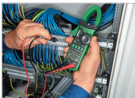
Voltage testing in switchgear cabinet
