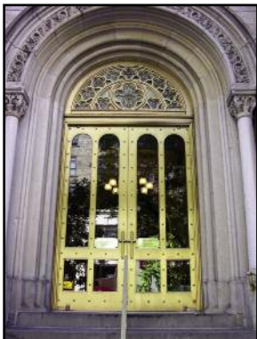
Marble Collegiate Church, NYC Renovation of Front Entrance
