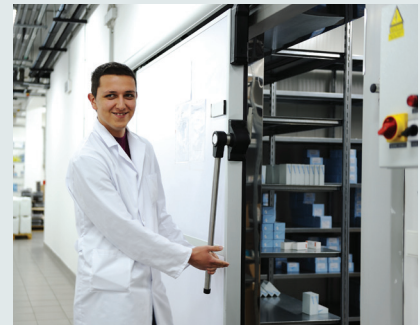
Walk-in Coolers and Freezers
