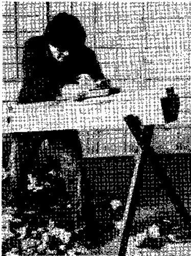
Shokunin [artisans] plane long materials using a pull stroke down an angled planing beam. Speed, a small blade angle, and holding the blade on a skew to the wood help the plane leave a smooth, highly polished surface.
