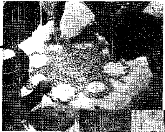
On the work site of the Royal Palace of Marrakesh: tile-setting, in reverse, a motif surrounding a twenty-four-pointed star.
