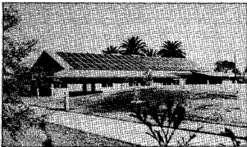
◀ The City of Dixon (California) recently dedicated this 20kW. photovoltaic energy system on top of the roof of their City Hall.
