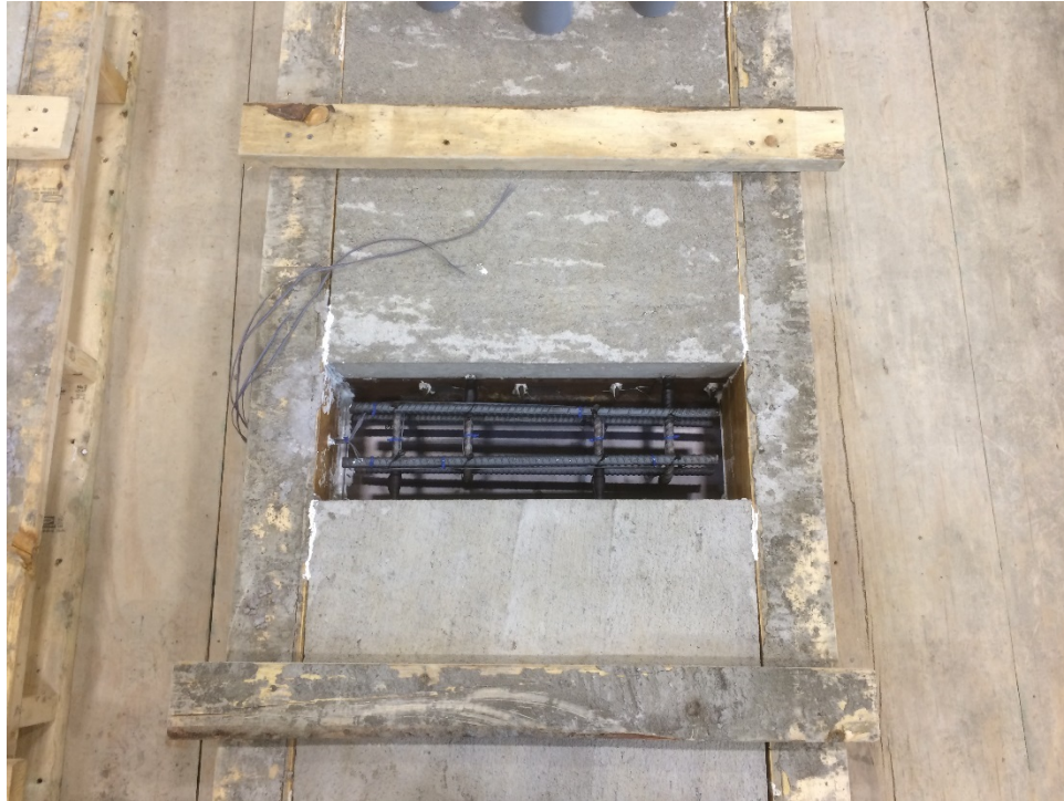
Figure 4.28 Joint Formwork
