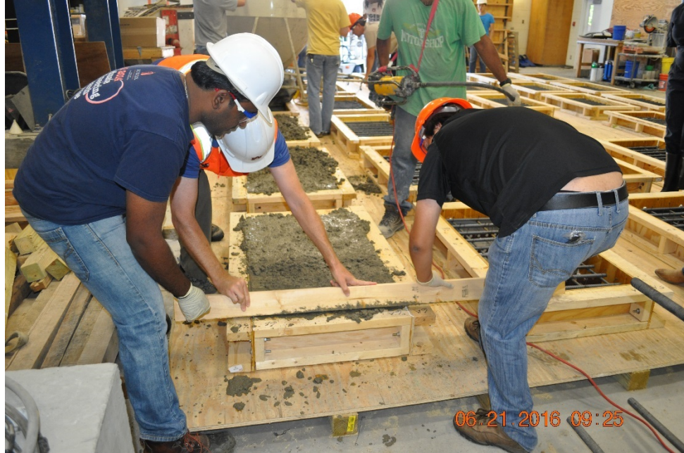
Figure 4.18 Screeding off the Excess Concrete
