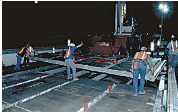
Figure 2.25 Tappan Zee Bridge Deck Placement (D.S. Brown Company 2017b)
