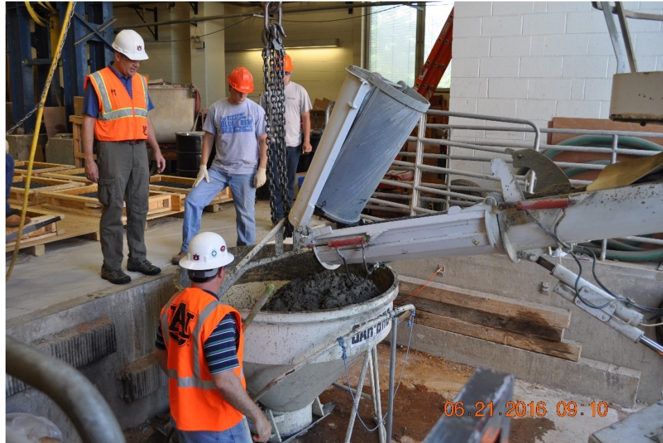
Figure 4.15 Delivery of Ready-Mixed Deck Concrete
