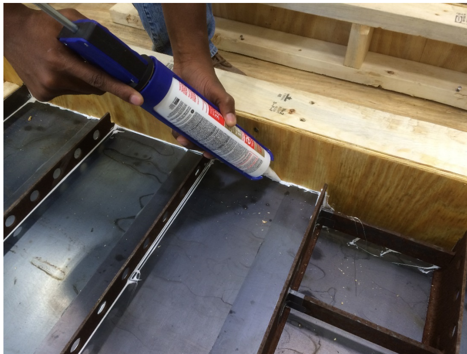
Figure 4.13 Caulking the Forms
