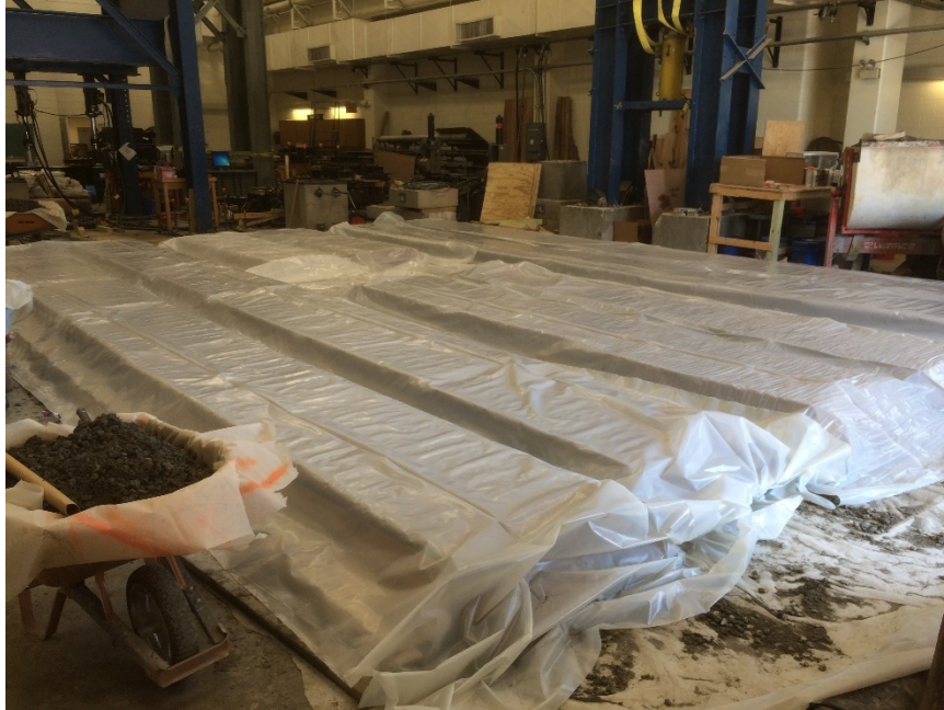
Figure 4.21 Wet Burlap and Plastic Sheeting over Panels
