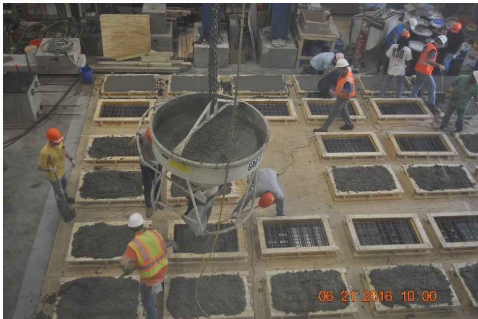
Figure 4.19 Overview of Concrete Placement
