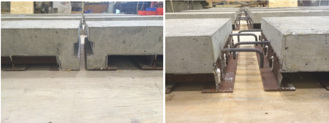
Figure 4.24 Close-up View of Panels before Grout Pour
