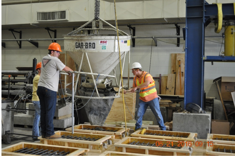
Figure 4.16 Placement of Concrete
