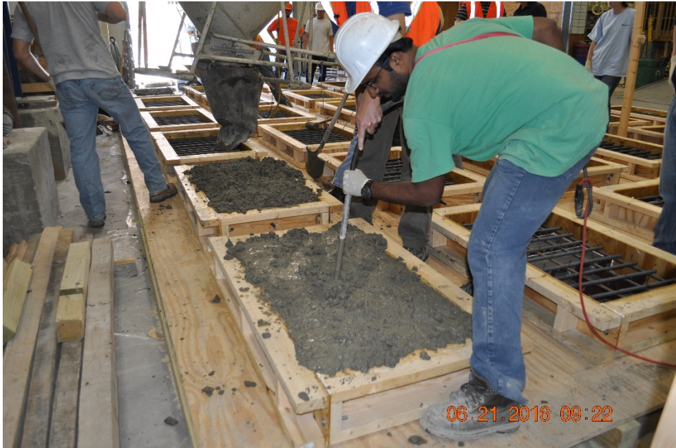
Figure 4.17 Vibrating the Concrete
