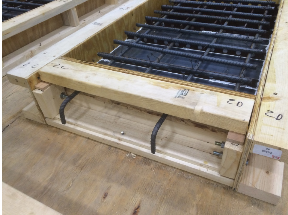
Figure 4.14 Close-up View of Completed Forms
