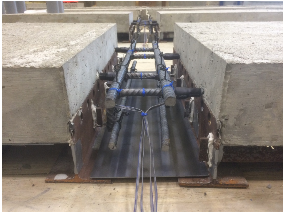
Figure 4.27 Protected ERSGs Mounted on Reinforcing Steel
