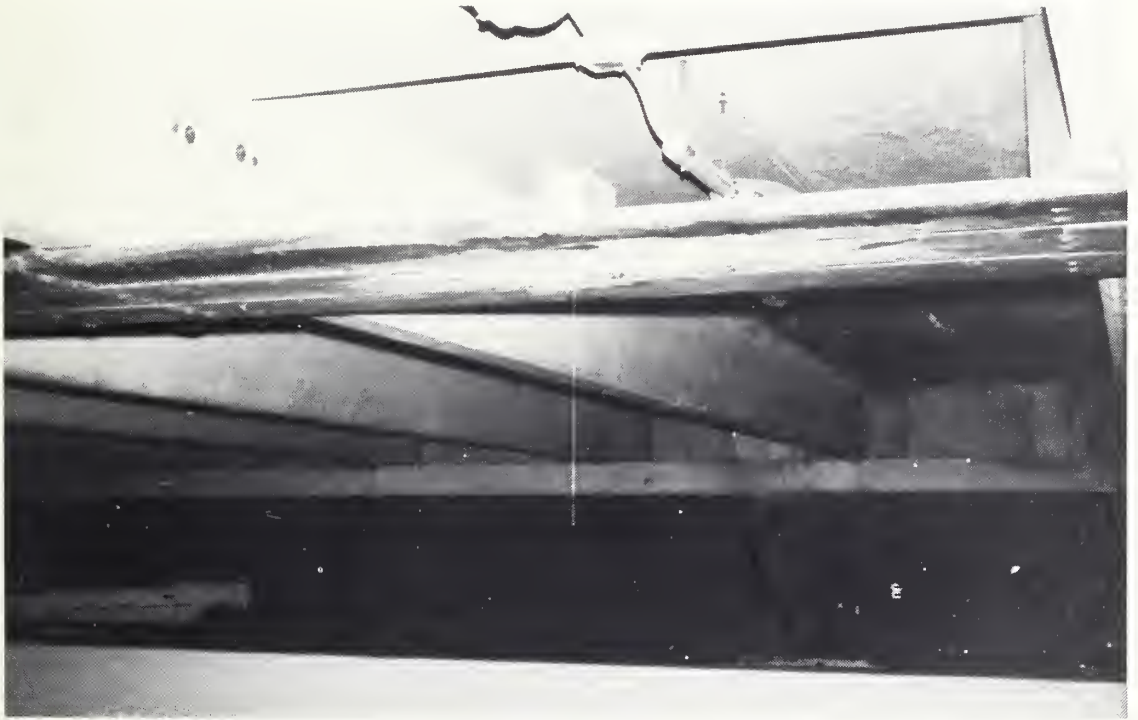
FIG. 9-2 SIGNPOST INSTALLATION IN 8TH STREET TUNNEL
