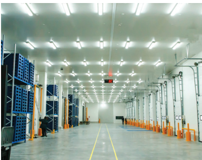
Cold Storage Warehouses
