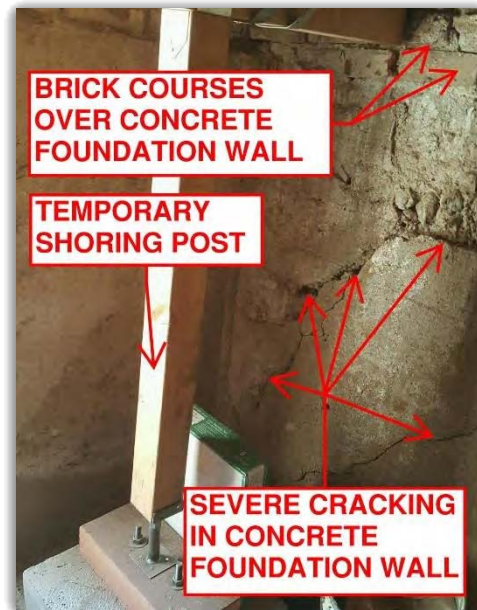
Figure 5 - Cellar Foundation Wall (July 27, 2016)
