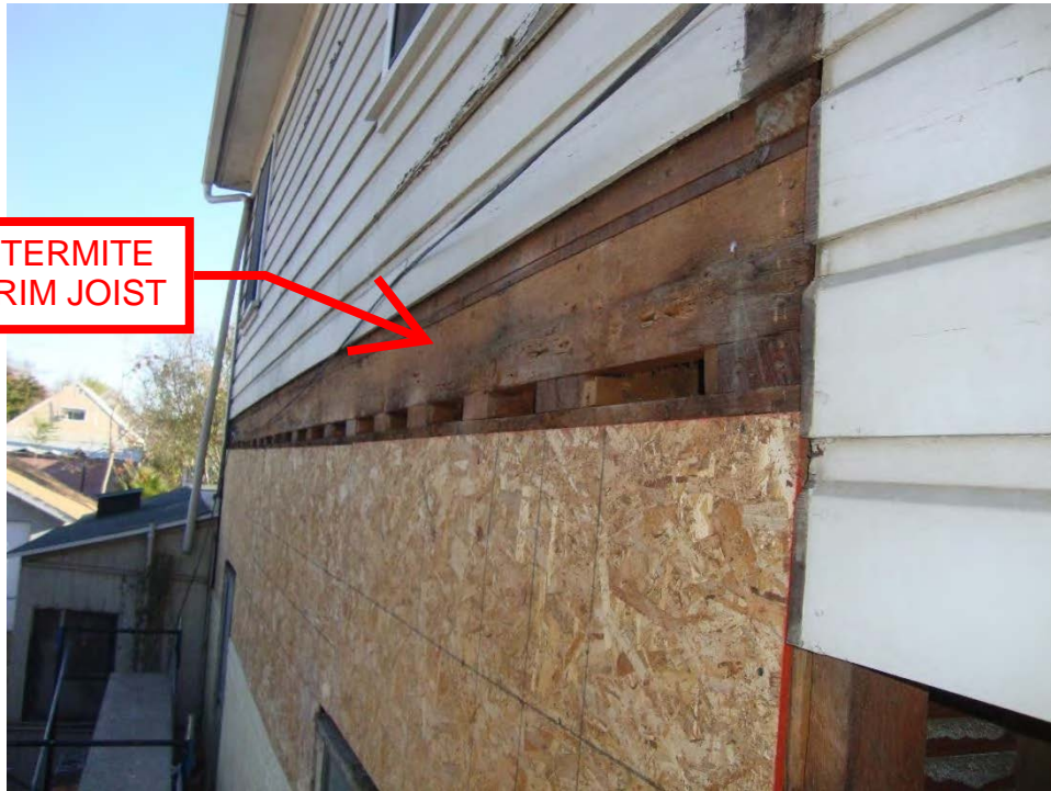
PHOTO 4: NORTH ELEVATION – 2ND FLOOR RIM JOIST
