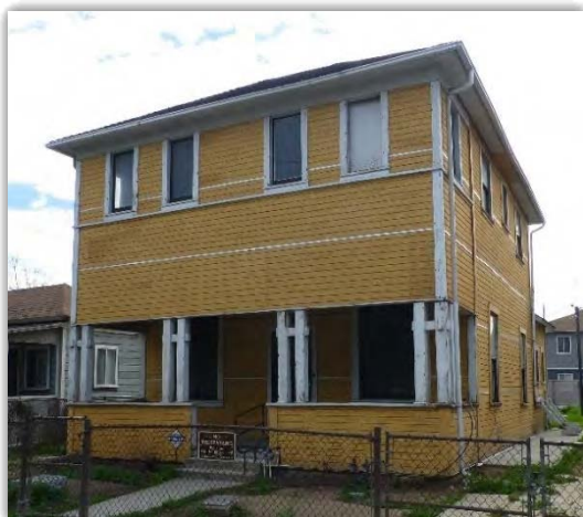
Figure 7: Harada House with Plywood Sheathing (March 20, 2018)
