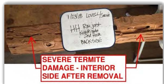
Figure 14 - Back side of Second Floor rim joist after being removed (January 23, 2018)
