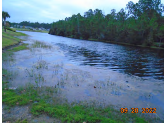
Pond J: Perimeter vegetation is decaying. Algae is forming around decay.
