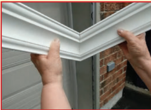
Create perfectly fitting interior crown molding joints
