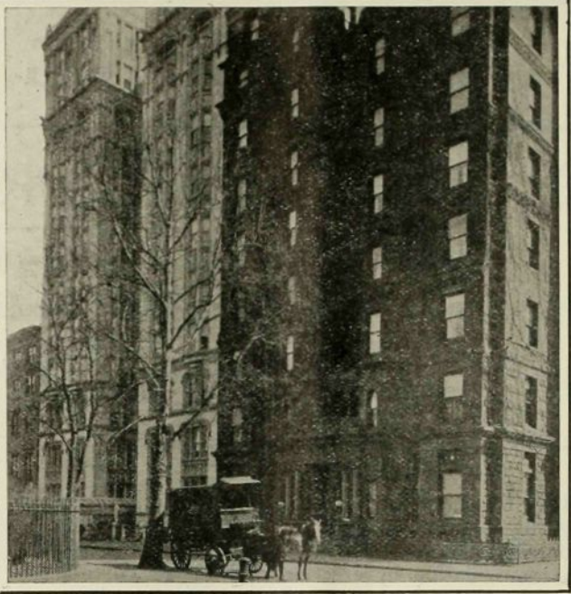
Showing the different appearance of the new Apartment Building to the left with wide court, built of light material and with plenty of window space. Contrast with building to the right with a narrow forecourt furnishing insufficient light to windows opening on it. Built of dark brick and stone. Gramercy Park, New York, N. Y.
