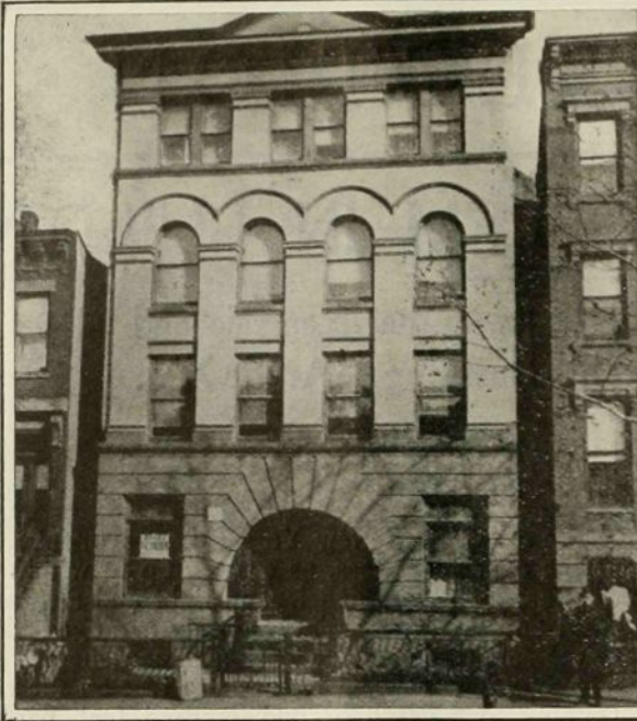
Over one-third of this frontage on ground floor occupied by an unnecessarily wide entrance, sacrificing accommodations and light of apartments. Less than one-third is used for windows. Eighteenth Street, Brooklyn, N. Y.
