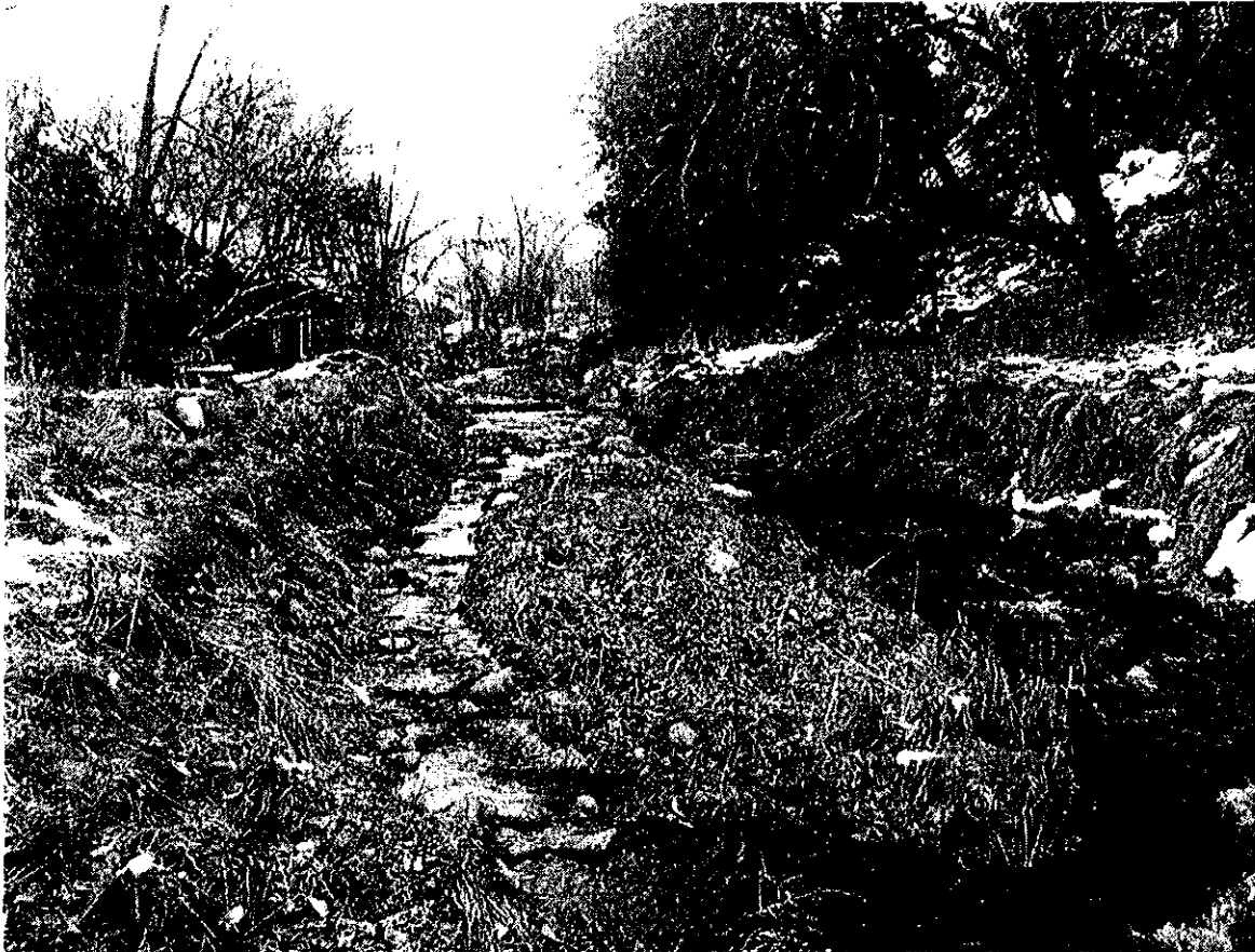
Drainage Basin 1 Channel
