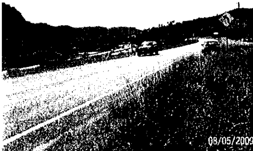
Looking westbound at MP 109.8
