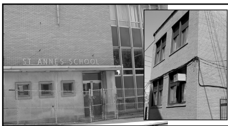
Saint Anne's Annex Jersey City • 7,000 sf
