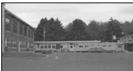
Nativity School Building, Midland Park • 14,800 sf
