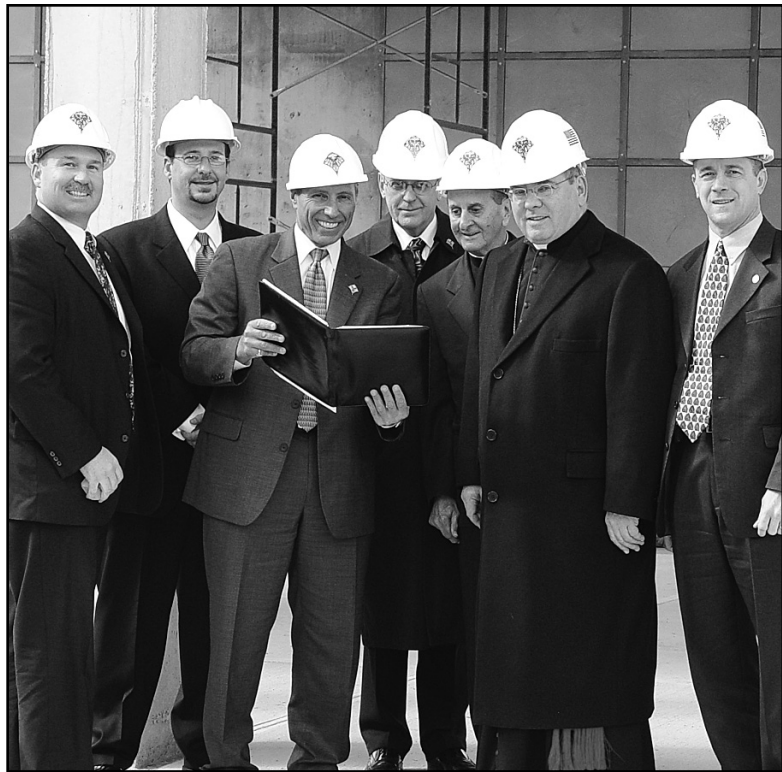
At the construction site of the new mausoleum are, left to right, Andrew Schafer, Robert Albert, Joseph Verzi, Richard Finan, Msgr. William Naedele, Archbishop John J. Myers and Deacon Joseph Dwyer.
