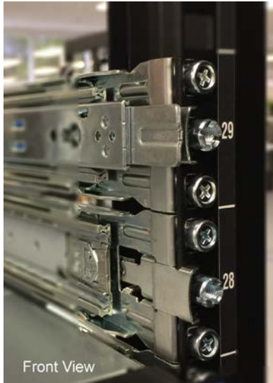
Figure 3-41. Rail attaching to front vertical rail
