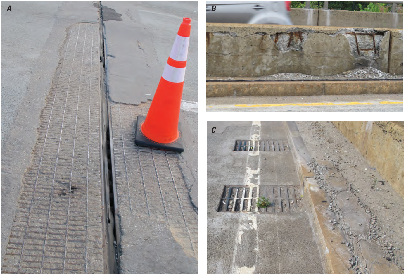
Figure 18. Sediment sources from deterioration of the A , bridge-deck surface; B , median barrier; and C , shoulder area that contributed to the sediment yield on the Interstate 90 bridge near Weston, Massachusetts, 2015–16. Location of bridge is shown on figure 1.
