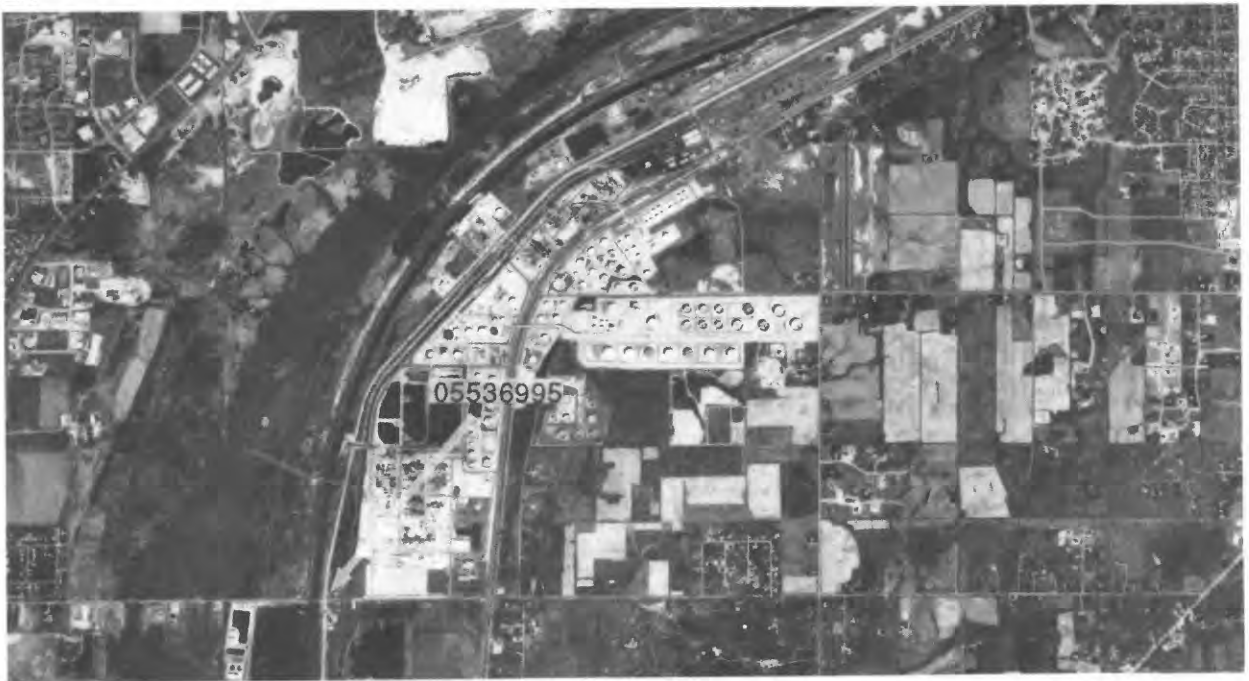
Figure 6.--Aerial photographs of (A) Des Plaines River at Riverside, Ill. (05532500), and (B) Chicago Sanitary and Ship Canal at Romeoville, Ill. (05536995), taken April 30, 1988, and April 17, 1988, respectively.
