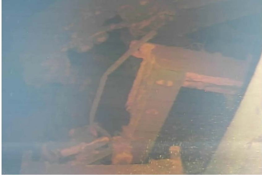
Figure 58. Image of relocated CRD rail on the 1F3 platform with no grating; obtained on July 19, 2017 (Courtesy of TEPCO Holdings [209]).
