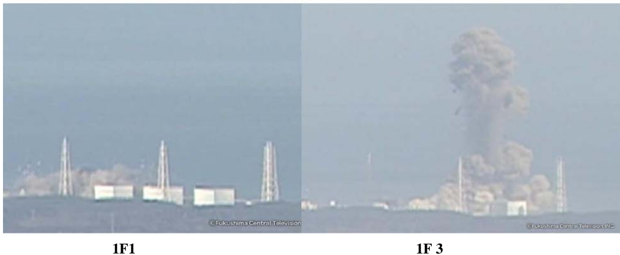
Figure 82. Images of 1F1 explosion compared with 1F3 explosion. (Courtesy of FCT [221])
