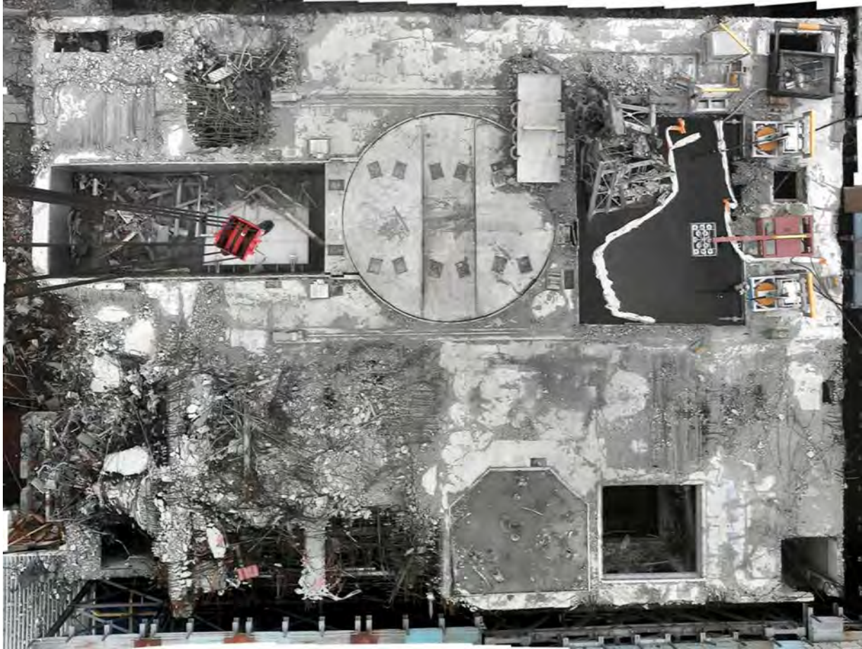
Figure 74. Damaged areas on 1F3 reactor building floor. (Courtesy of TEPCO Holdings [16])
