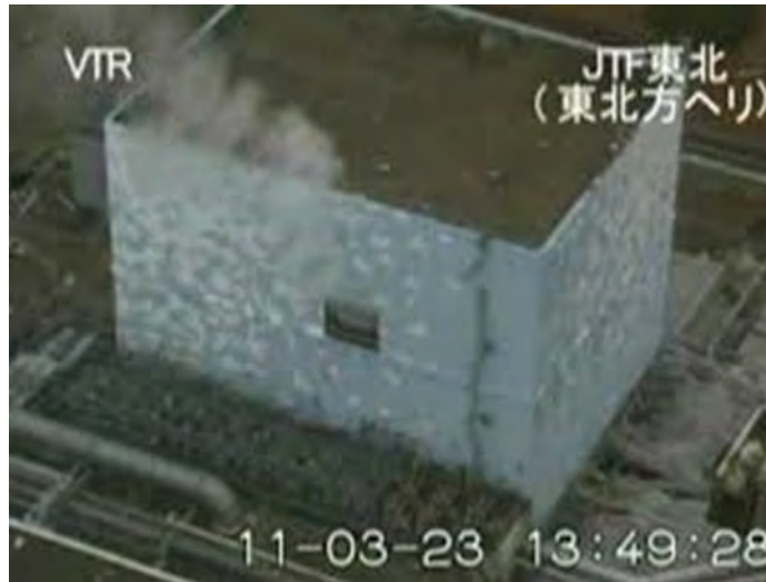
Figure 27. 1F2 reactor building with open blowout panel. (Courtesy of TEPCO Holdings [185])
