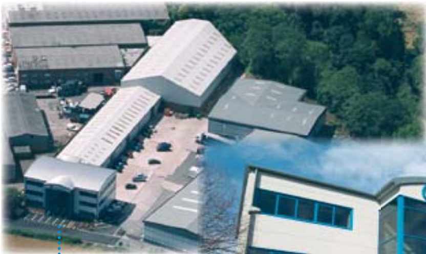
Cembre Ltd. factory in Curdworth (Birmingham)
