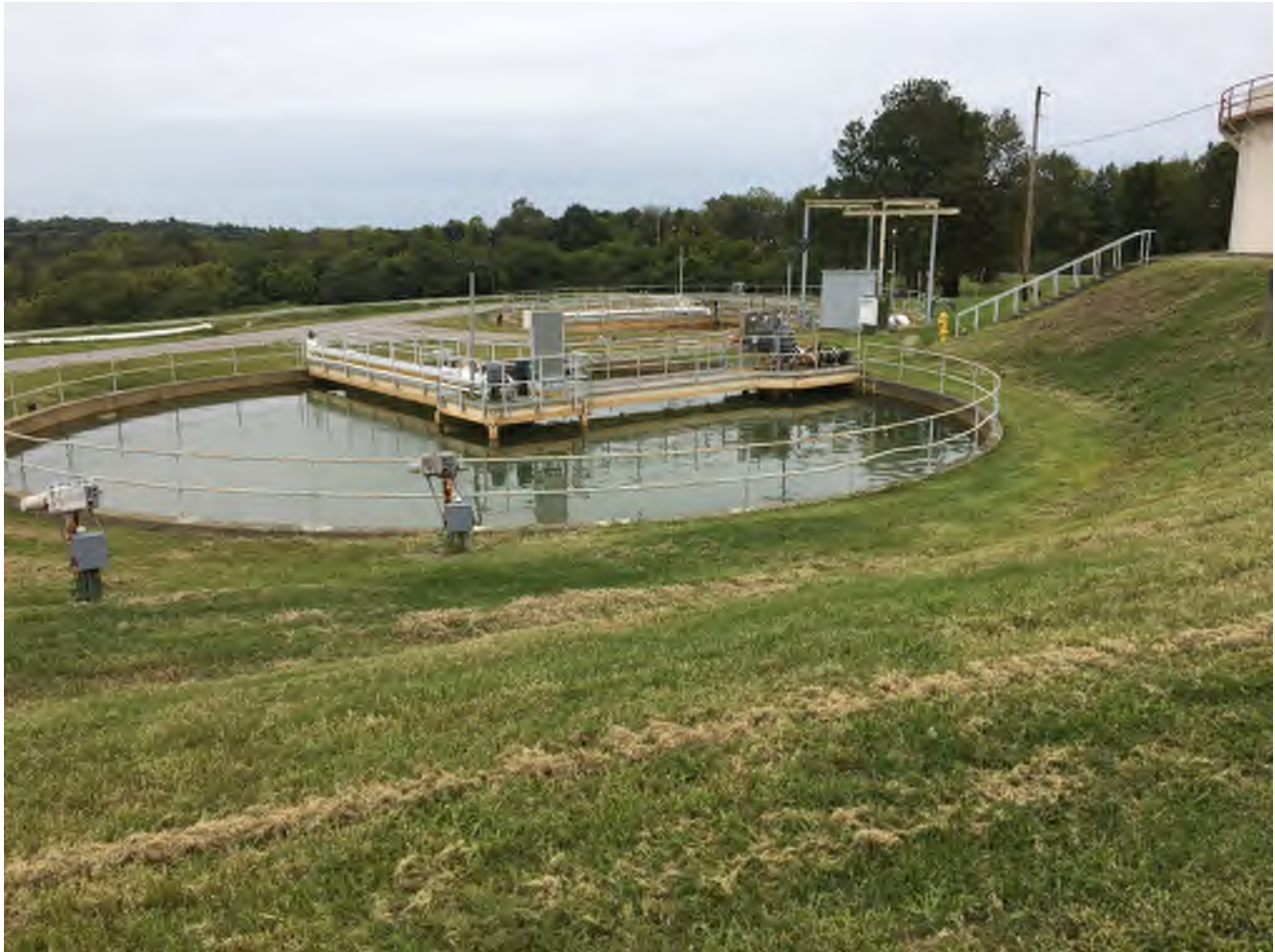
Figure 6. Photograph of WWHTs and Electrical Cabinet (next to staircase)
