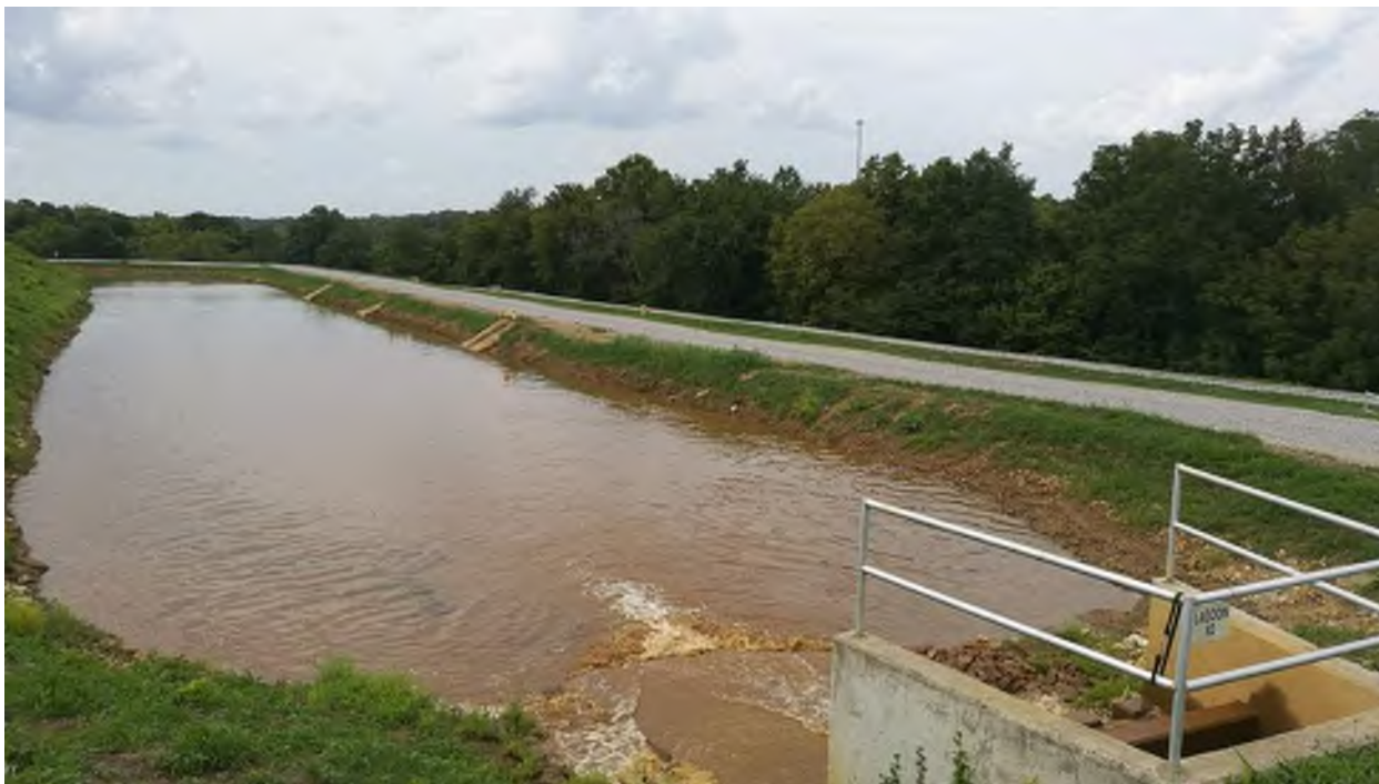
Photo 3: Washwater Discharge to Lagoon No. 2
