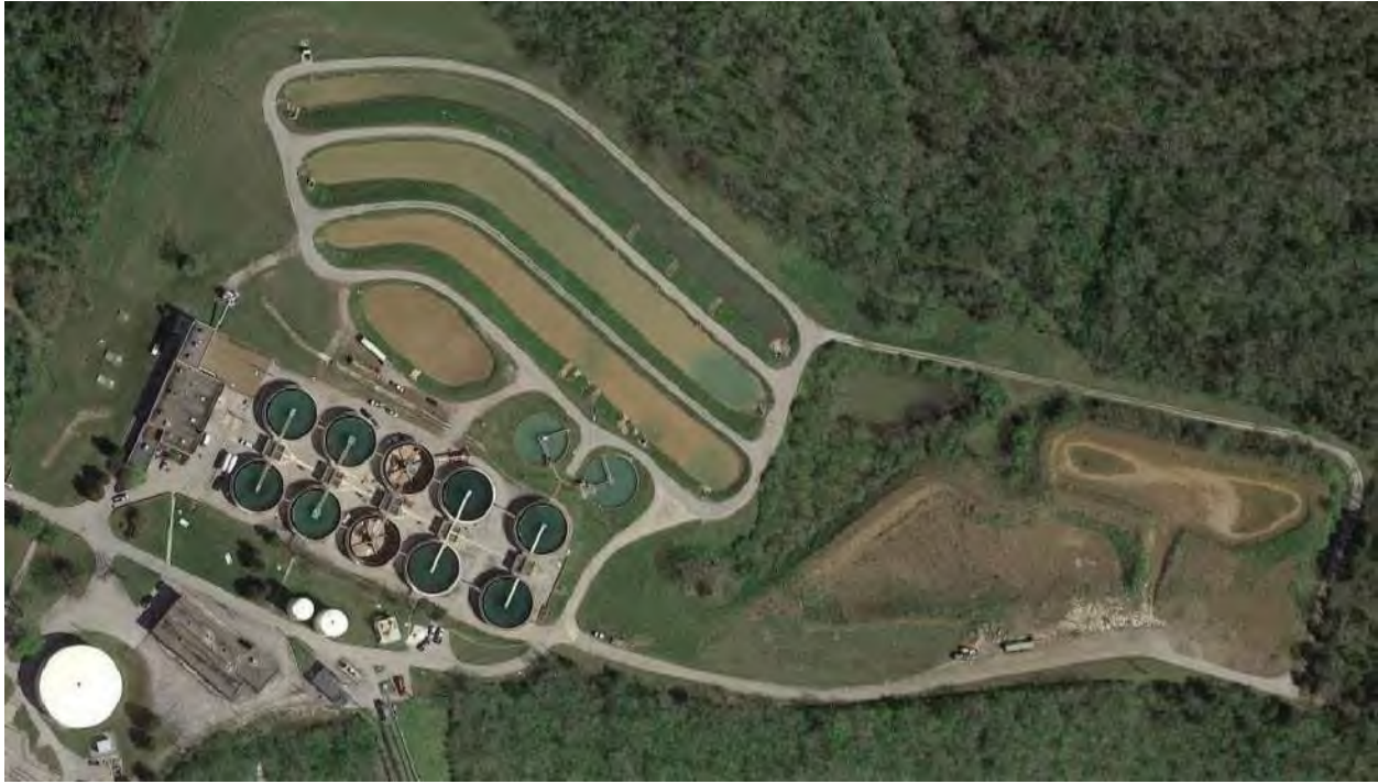
Figure 1. Existing KRS1 Water Treatment Plant
