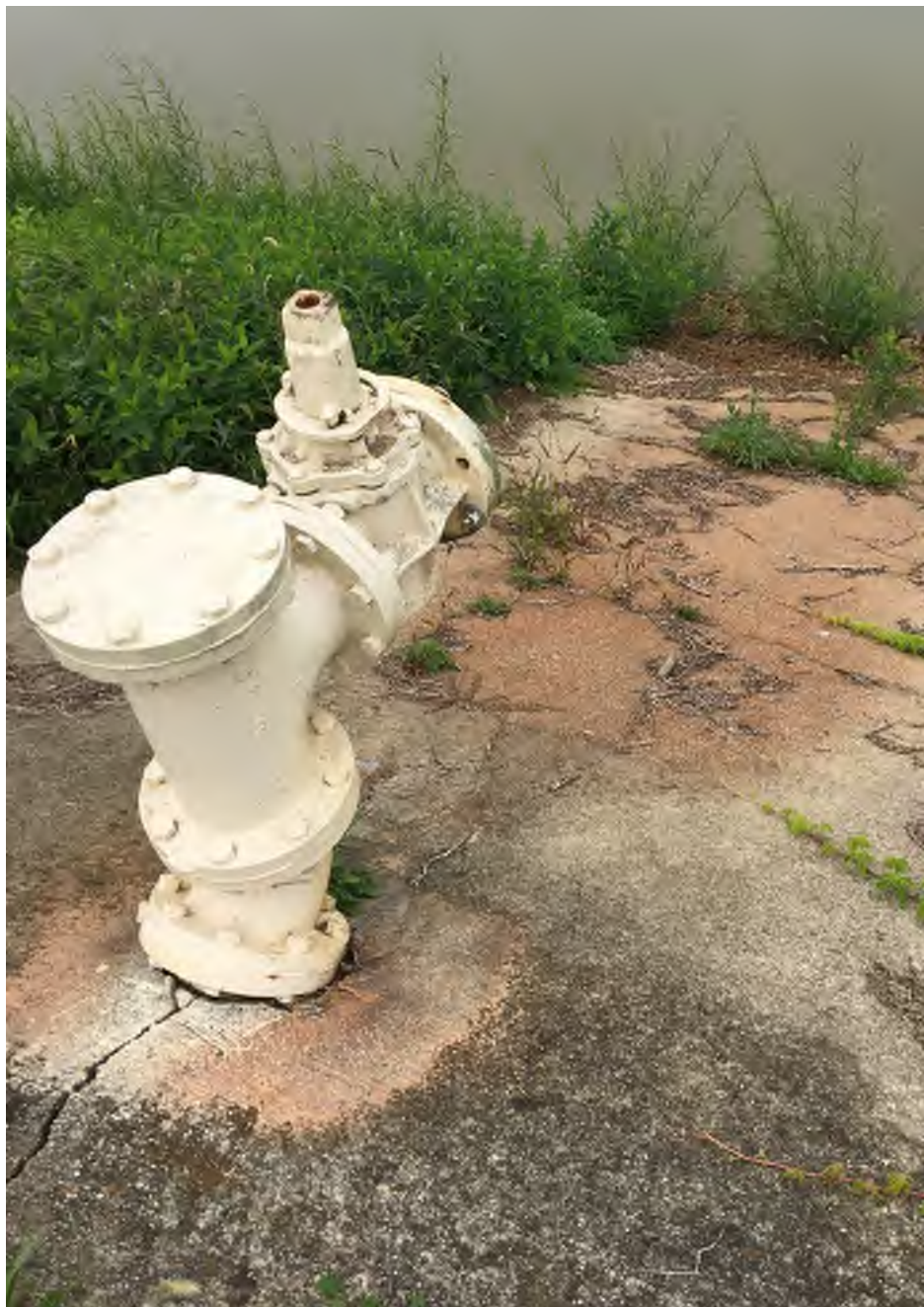
Figure 7. Photograph of 6-inch Sludge Force Main Connection
